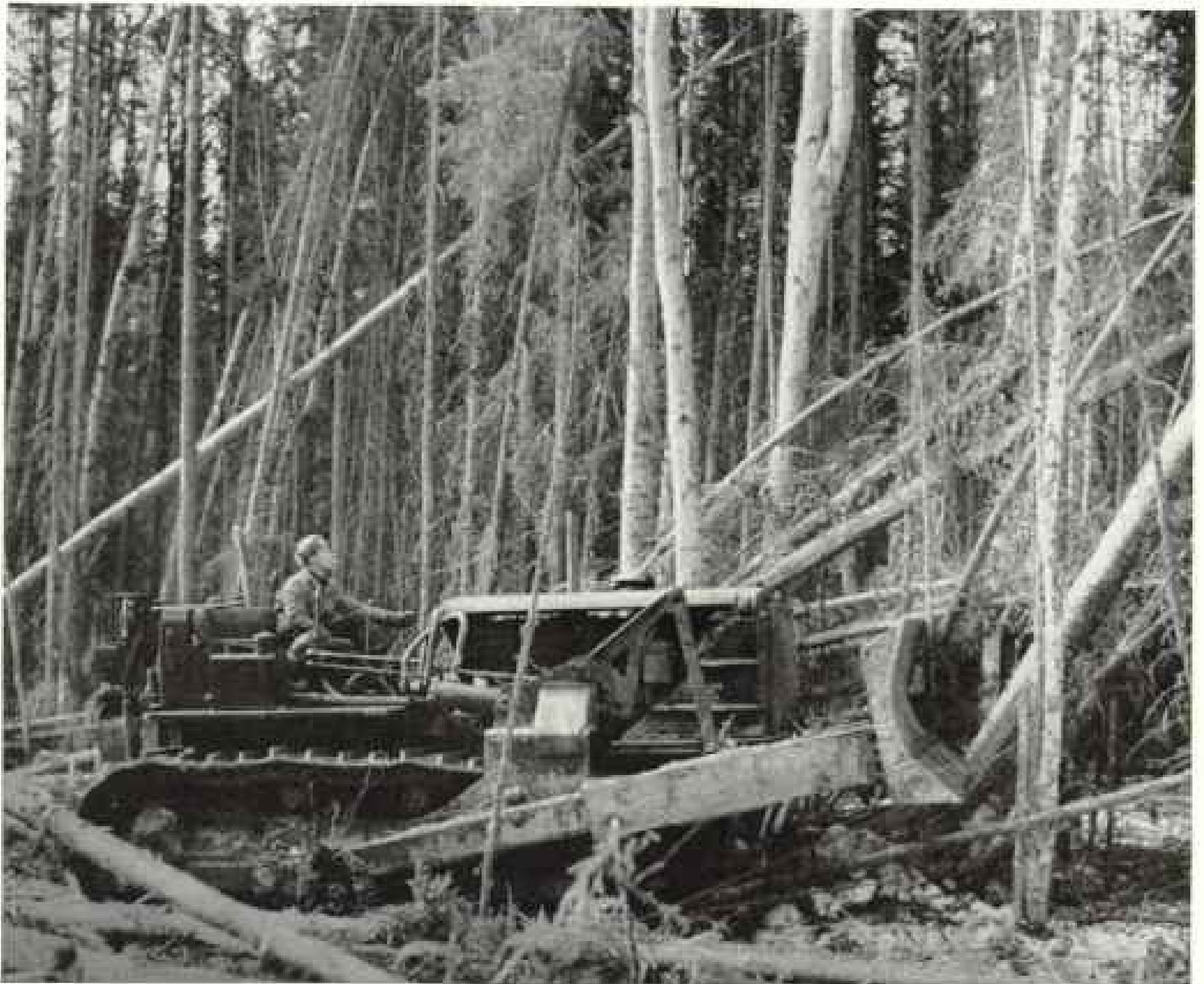
U. S. Army Engineers
