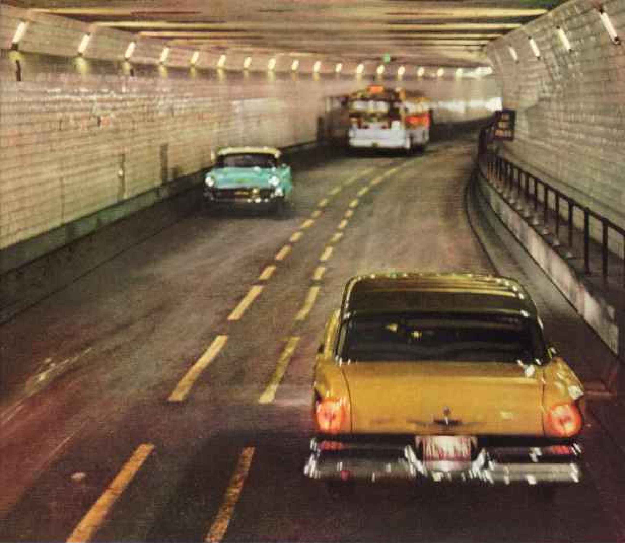
The Detroit-Windsor tunnel is one mile long—with 2200 feet of its length directly under the Detroit River.
