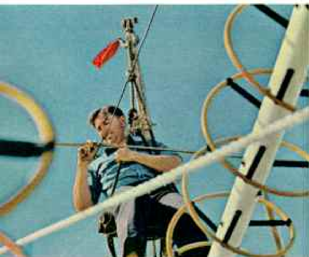
Block and tackle hoist an Aussie technician aloft to repair spiral antennas on a Muchea transmitter.
