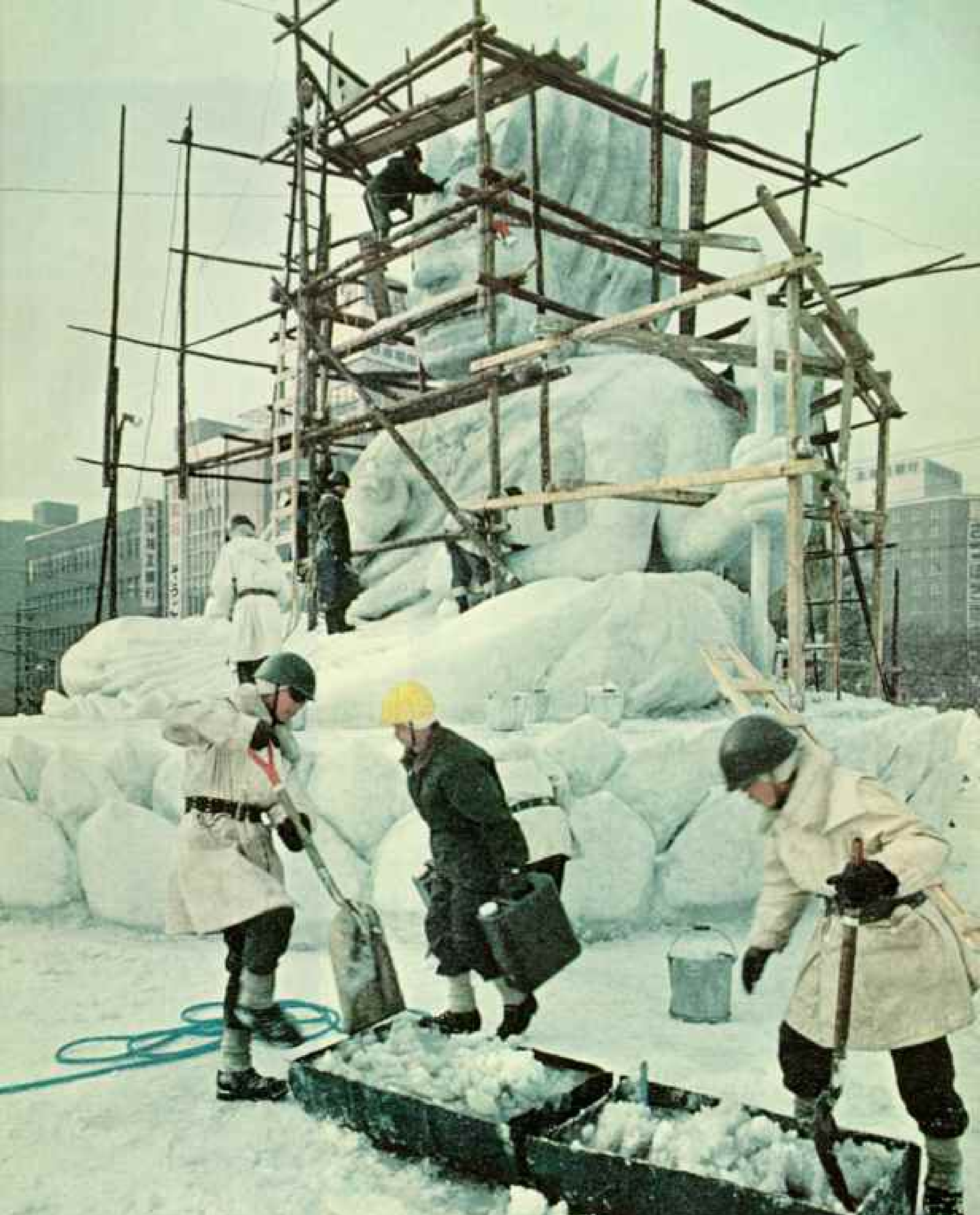
FIERCE FIGURE of Aizen Myo-o, the Buddhist god of love, emerges from a platform of snow. Soldiers stir "cement"—a quick-freezing mixture of snow and water used to mold and shape the deity's features. Temporary scaffolding gives shaky support to carvers.
