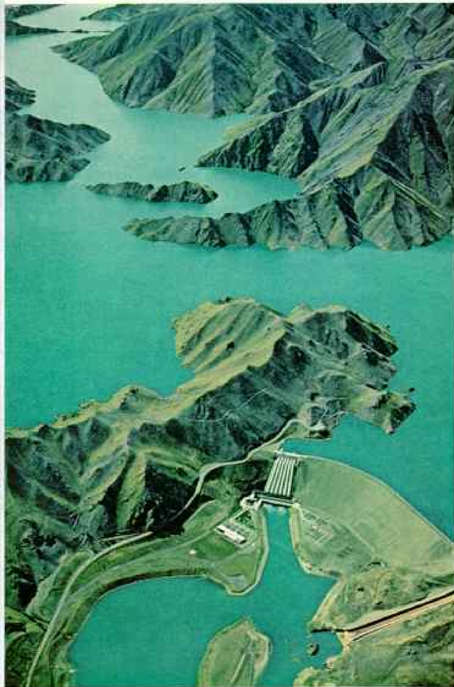
Largest man-made lake in the nation, azure Benmore spins hydroelectric turbines at the foot of its earthen dam, providing 540,000 kilowatts of energy. Power flows to the North Island by cable under Cook Strait.
