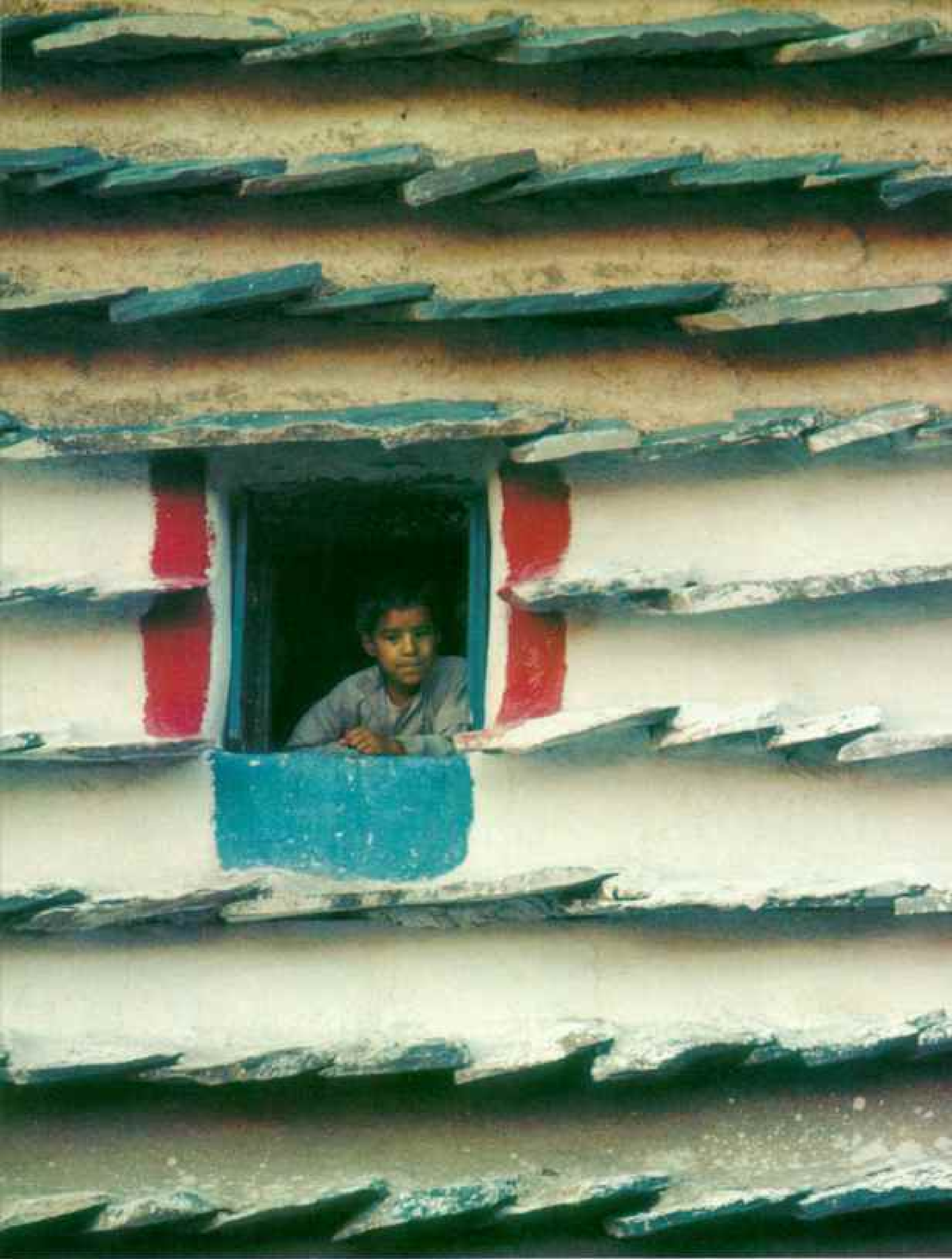
Time-honored and practical, the layered architecture typical of Asir Province is counterpointed by a television antenna wire. Slate shelves deflect rain from the
