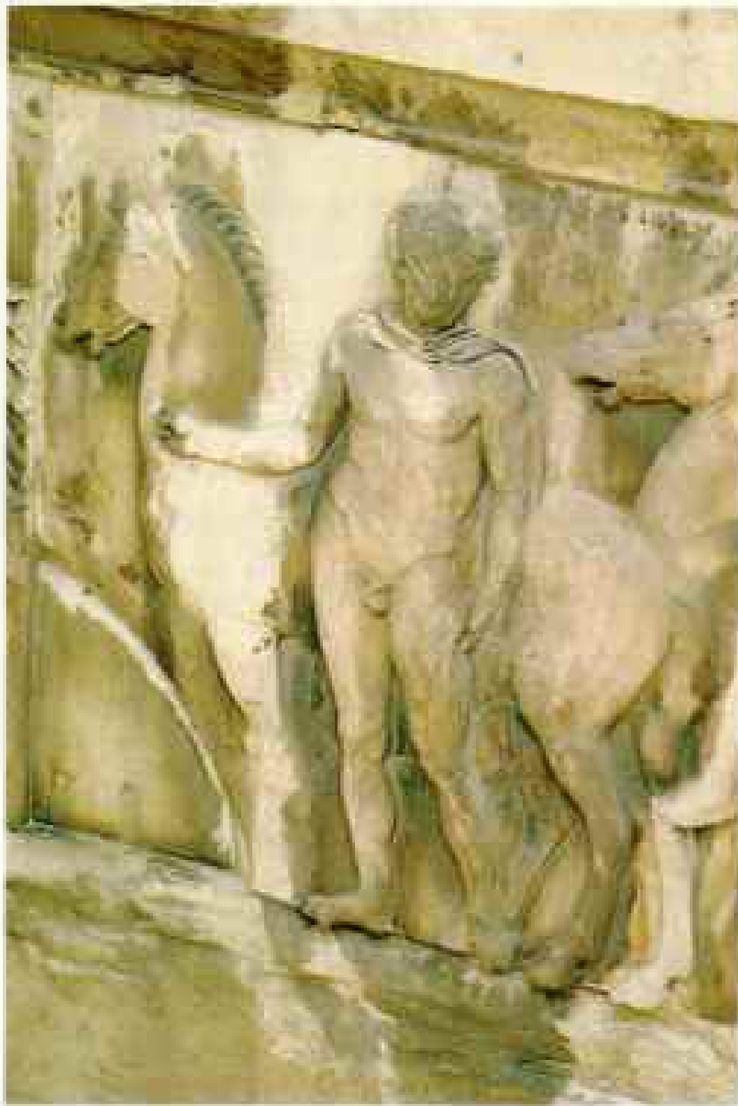
Erasing the beauty of classical Greece, sulfur oxides in the smog over Athens chemically transform marble into gypsum, causing it to crack and flake off. A frieze panel on the Parthenon (left) has lost much of its detail, compared with another panel (right) preserved at the British Museum since the early 19th century.
