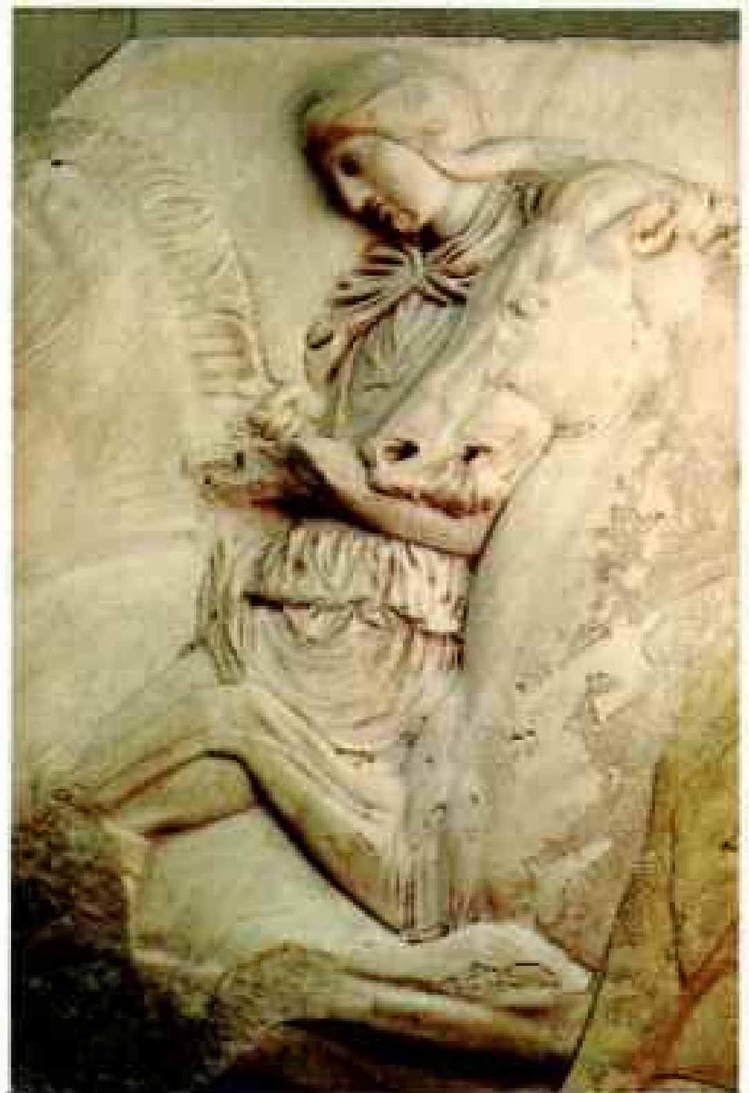
Erasing the beauty of classical Greece, sulfur oxides in the smog over Athens chemically transform marble into gypsum, causing it to crack and flake off. A frieze panel on the Parthenon (left) has lost much of its detail, compared with another panel (right) preserved at the British Museum since the early 19th century.
