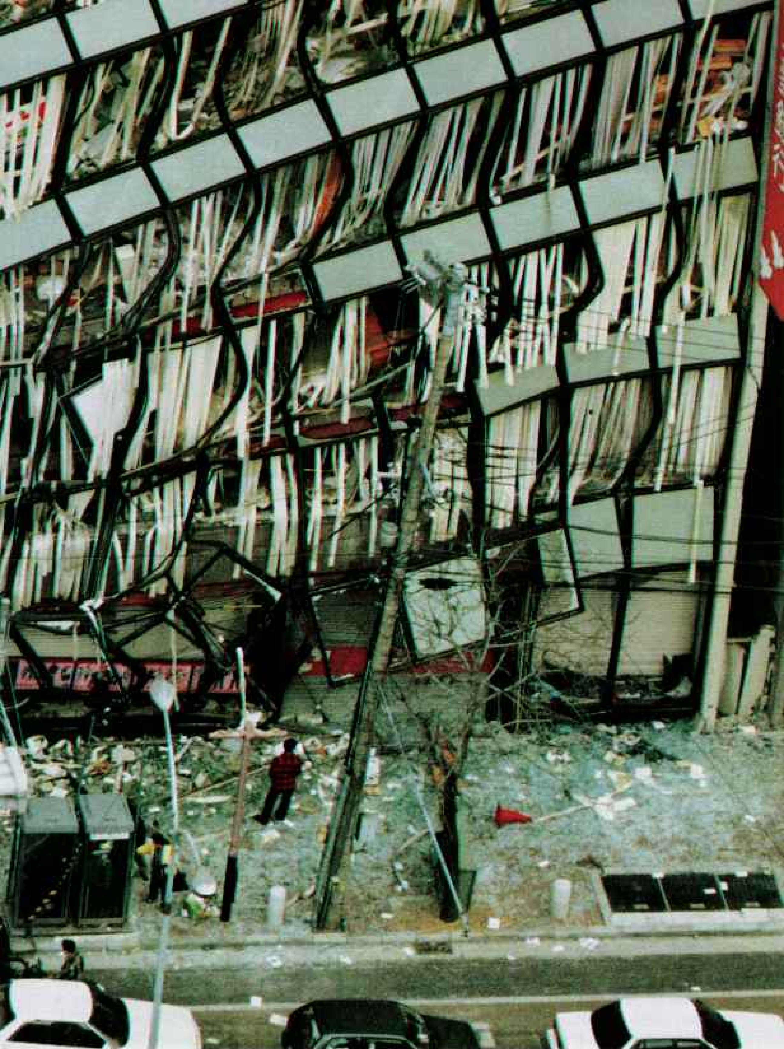
Sited on a filled estuary, the drooping structure illustrates the danger of erecting high-rise buildings on soft, unstable soil in a region prone to seismic action.
