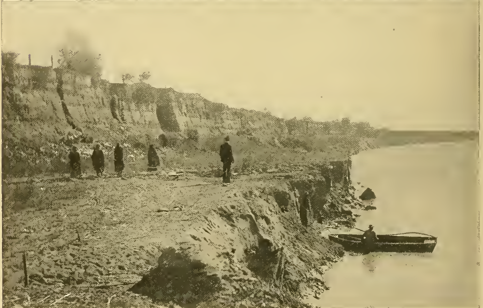
END OF THE PROTECTIVE LEVEE AT THE INTAKE OF THE IMPERIAL CANAL SYSTEM BELOW YUMA. CUT THROUGH AND DESTROYED BY THE COLO- RADO RIVER IN DECEMBER, 1906
