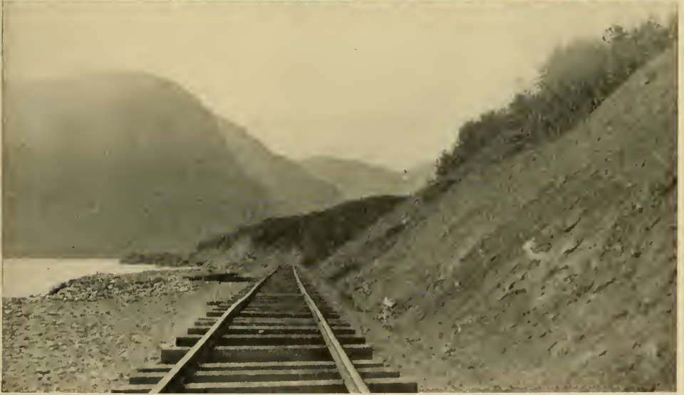
A SHARP CURVE IN THE RAILWAY AT ABERCROMBIE RAPIDS: A NARROW SHELF BLASTED OUT FOR THE ROAD
