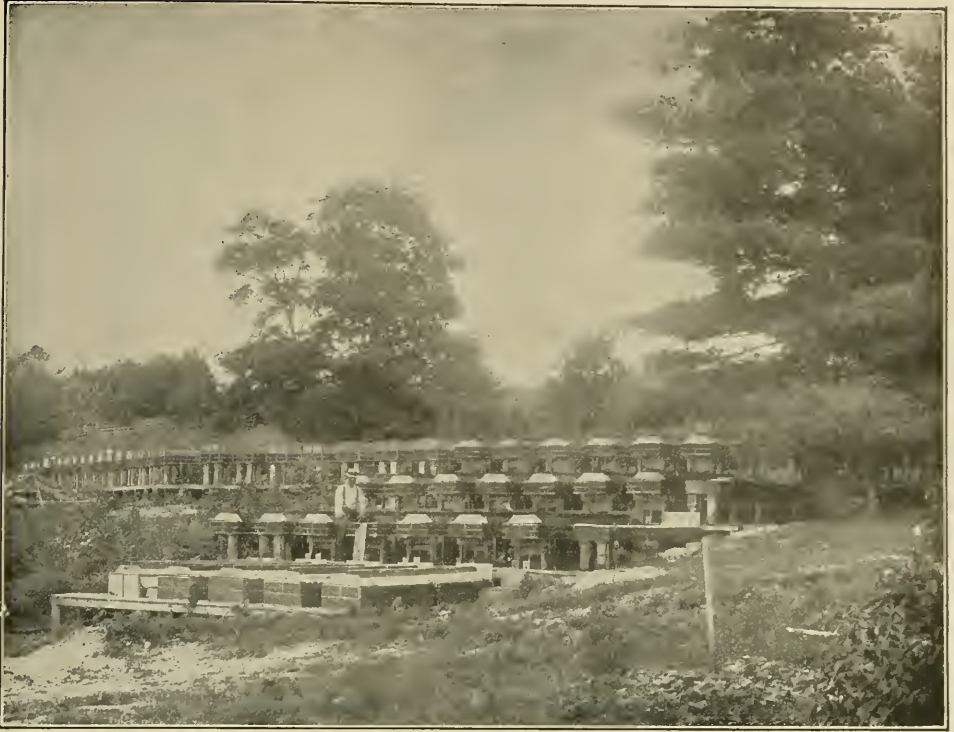
OPEN-AIR TROUGHS FOR REARING SALMON AT A HATCHERY ON THE PENOBSCOT RIVER IN MAINE (SEE PAGES 432 AND 433)
