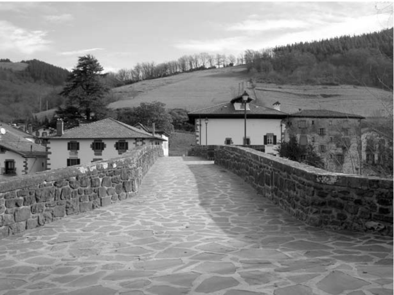
Fig. 16b. The bridge at Sumbilla, seen from above. (Photos by author 2004)
