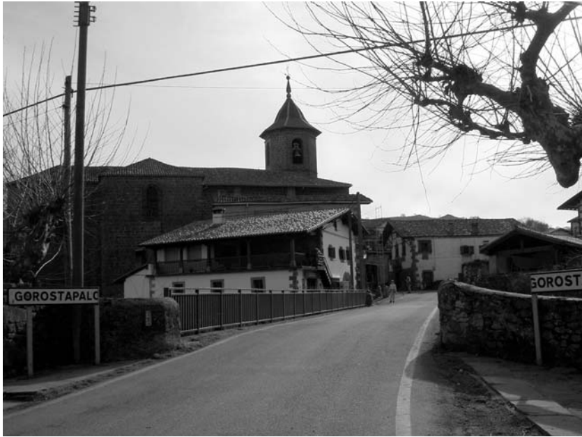
Fig. 19. The Stone Bridge in Errazu with the church in the background. (Photo by author 2004)
