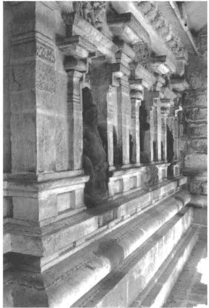
Fig. 32. Niches housing (from left) Agastya, Śiva Naṭarāja, and Gaṇeśa. South wall of the ardhamaṅḍapa seen from the west, Āpatsahāyeśvara temple, Āḍuturai. Indentation at juncture with the vimāna is visible at far left.
