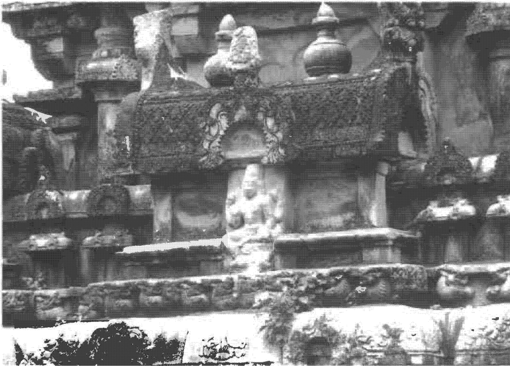
Fig. 30. Attached half-columns flanking the central aedicula of the superstructure (upper corners of photograph), Ghṛitasthāneśvara temple, Tillaisthānam.
