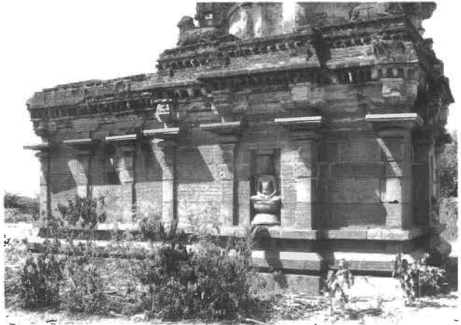
Fig. 25. Ground-level walls of the Kadambavaneśvara temple, Ērumbūr. Built by Iruṅgōlan Gunavaṇ Aparājitaṇ in 935. Seen from the north. The vimāna is to the right and the ardhamaṇḍapa to the left.
