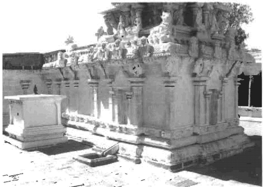
Fig. 34. Main walls of Tiruttoṅḍiśvara temple, Tirunāmanallūr. Built by Queen Kōkkiḷāṇ before 935. Seen from the northwest. The vimāna is to the right and the ardhamandapa to the left.
