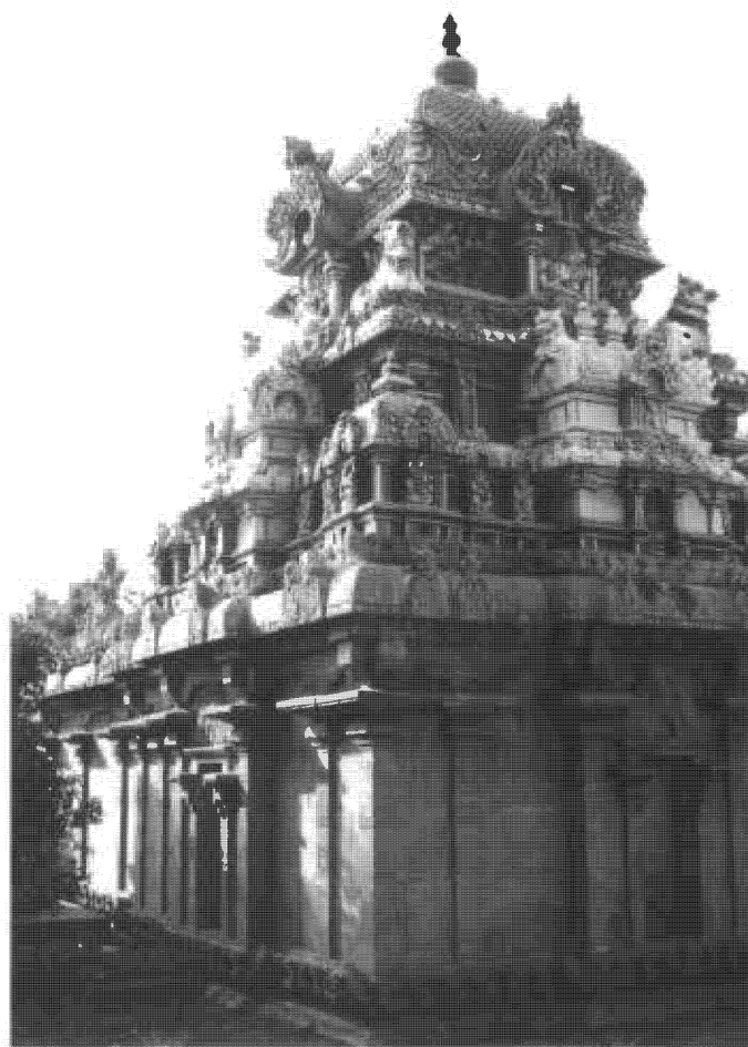
Fig. 1. Candraśekhara temple seen from the northwest, Tiruccendurai. Built by 908 by Naṅgai Bhūti Āditya Piḍāriyār (this and all succeeding photos by author).
