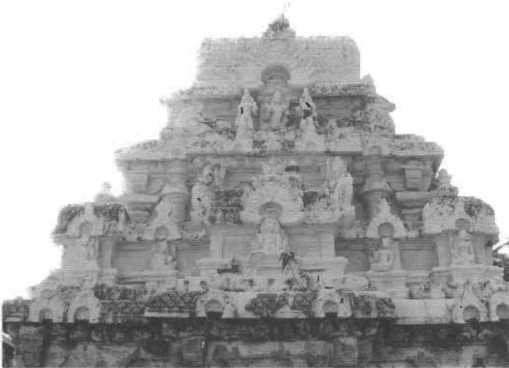
Fig. 29. Attached half-columns between the top and bottom tiers of the superstructure, and flanking the central aedicula (detail), Īdaneśvara temple, Tiruccātturai.
