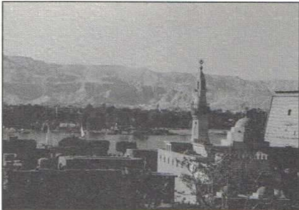
Fig. 44. Luxor, the Mosque in the foreground is located in the courtyard of the Luxor town temple. Theben West is across the Nile. In the background are the south-facing wadis that lead to the Valley of the Kings and the Valley of the Queens. Editor's photograph, 1989.
