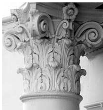
Capitol displaying four volutes, four flowers, and two ranks of acanthus leaves.
