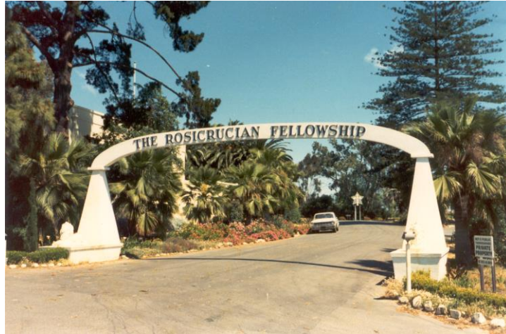
98. The new main gate.
