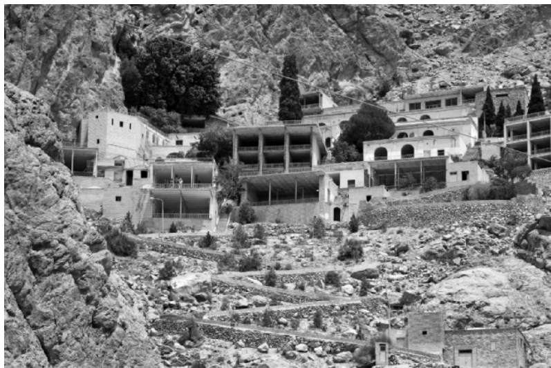
Fig. 24. Pir-e Sabz shrine and sheltered area for pilgrims, Yazd province, Iran.
