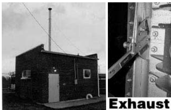
Execution Gas Chamber at the Mississippi State Penitentiary Note: High exhaust stack on Death House (left)
