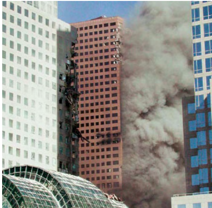
(b) WTC 7 , South Facade/Corner
