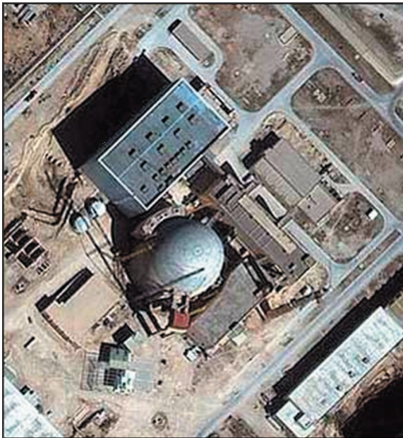
Figure 1. Bushehr Light Water Reactor.
