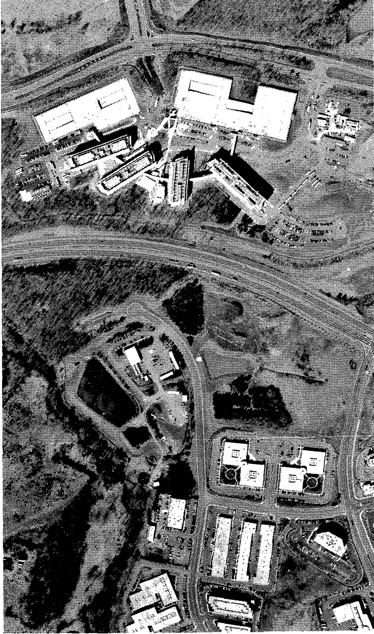
Aerial photo of the National Reconnaissance Office facility. © 1995 VARGIS, LLC. • All Rights Reserved.
