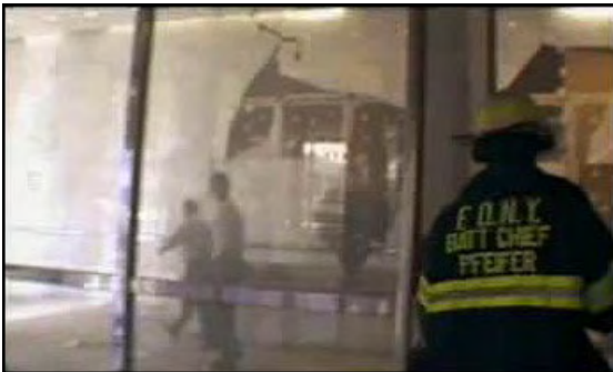
WTC lobby damage from underground blast – Naudett 9/11 Documentary
