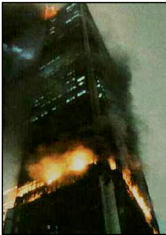
First Interstate Bank fire Los Angeles 1988
