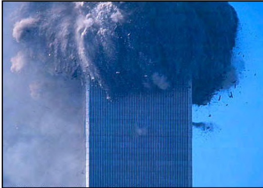
Demolition charge firing below the collapse
