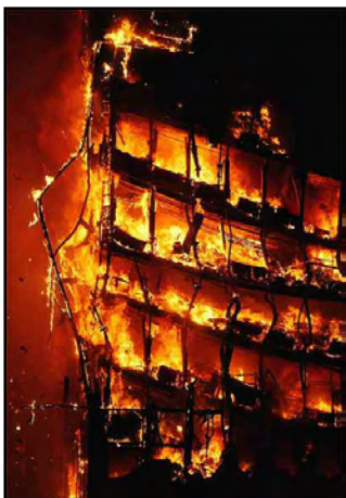
Windsor Building Fire Madrid Spain 2005
