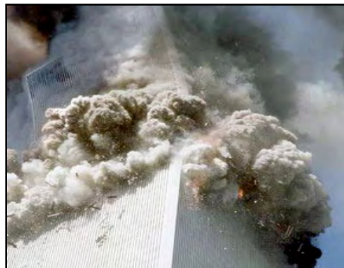
Top floors of WTC-2 leaning over the center axis almost 20° - notice the blast wave encircling the building
