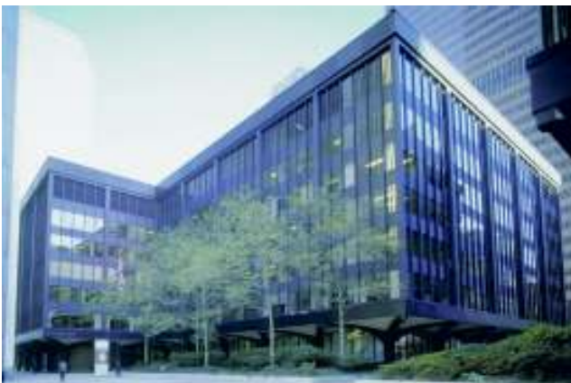
Building 6 of the World Trade Center
