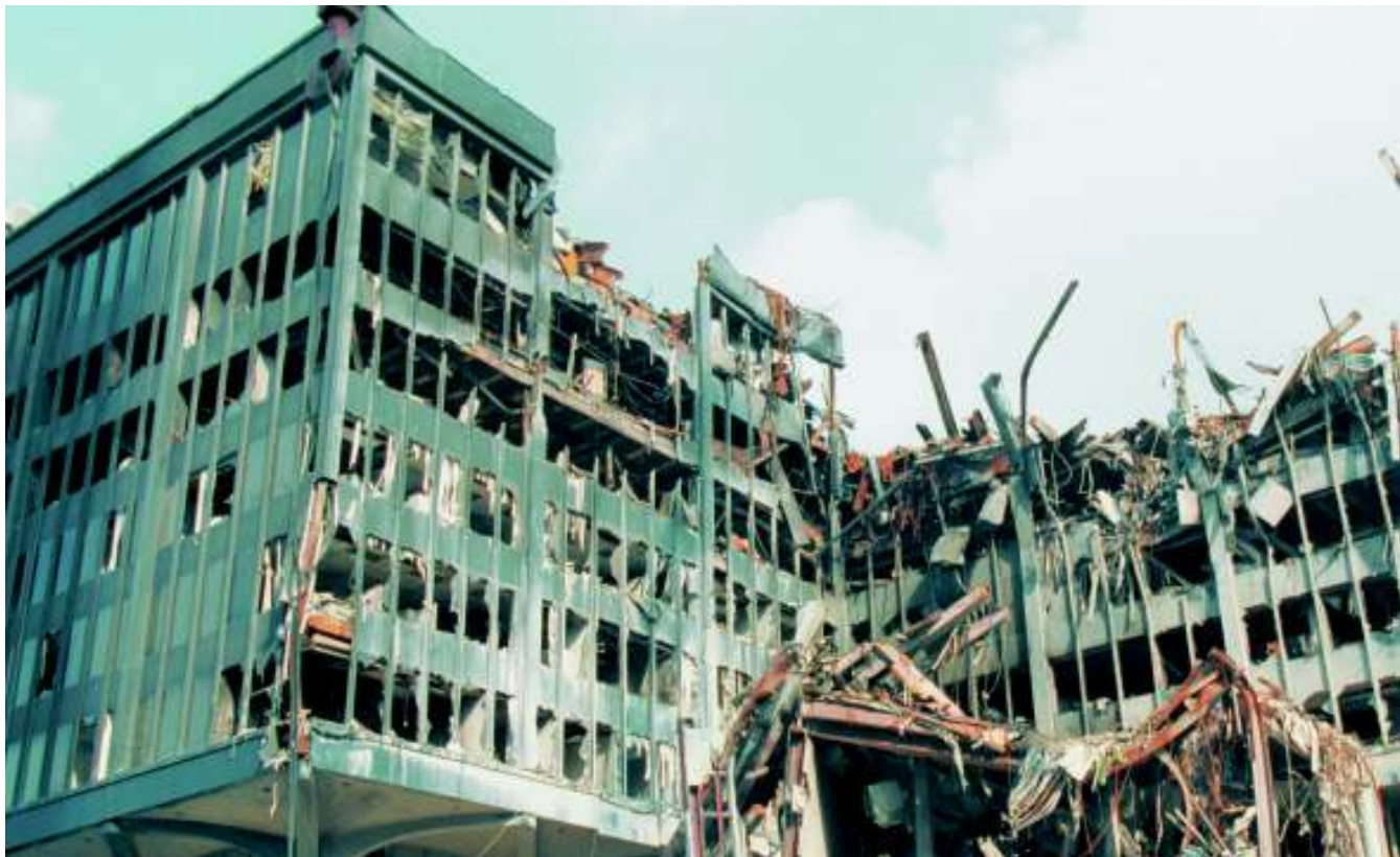
Figure 6-3 Building 6 survived the intense fires without crumbling. The debris from the tower crushed some of this building; the fire did not do that damage. (See Figure 6-4 to understand what this photo shows.)
