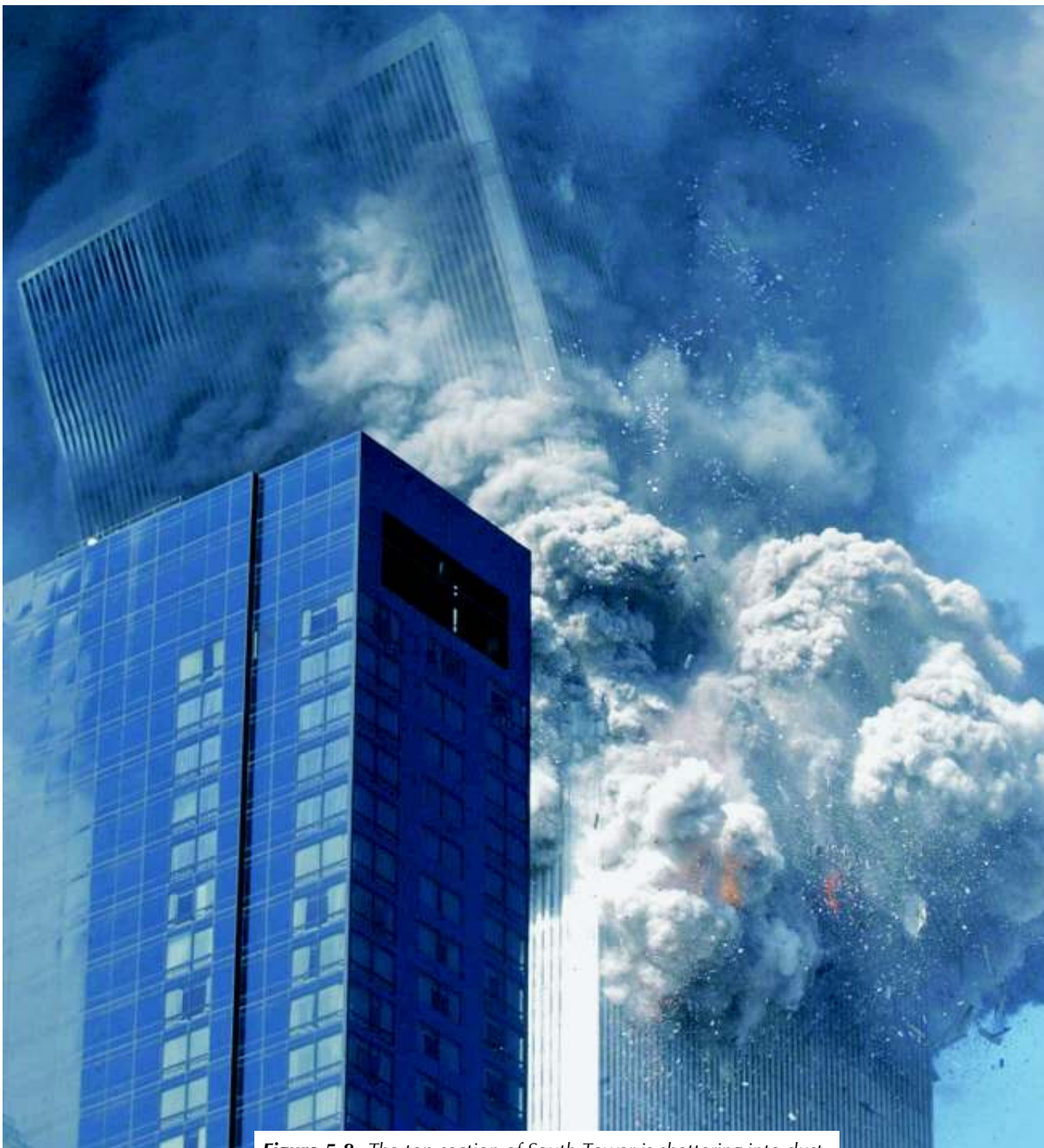
Figure 5-8 The top section of South Tower is shattering into dust
