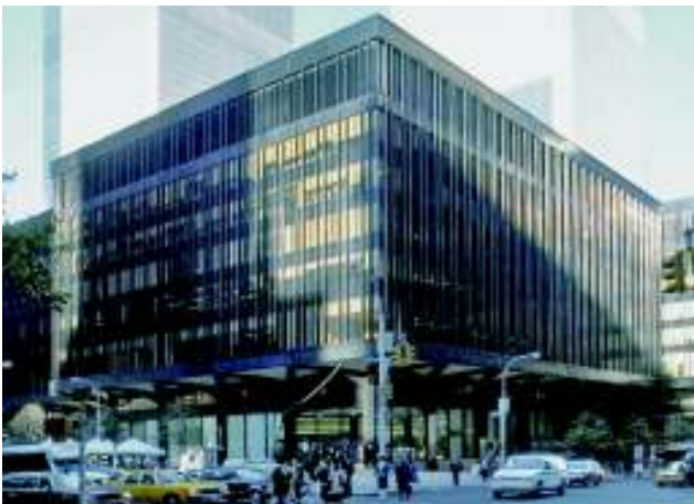
Building 5 of the World Trade Center
