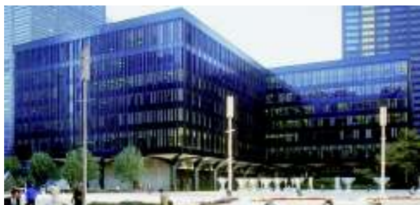
Building 4 of the World Trade Center
