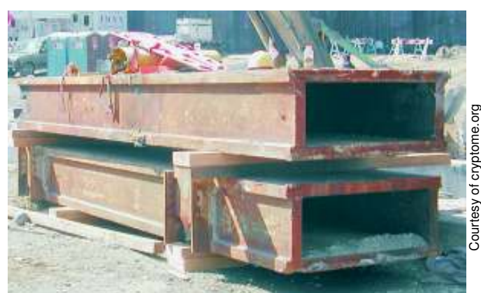
Figure 3-6 Core columns, sliced and ready to sell as scrap. This photo was taken at the WTC on October 3rd, 2001.
