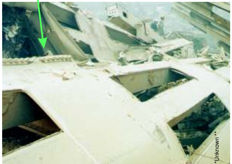
Figure 3-11 The bolts holding the pre-fab units together.
