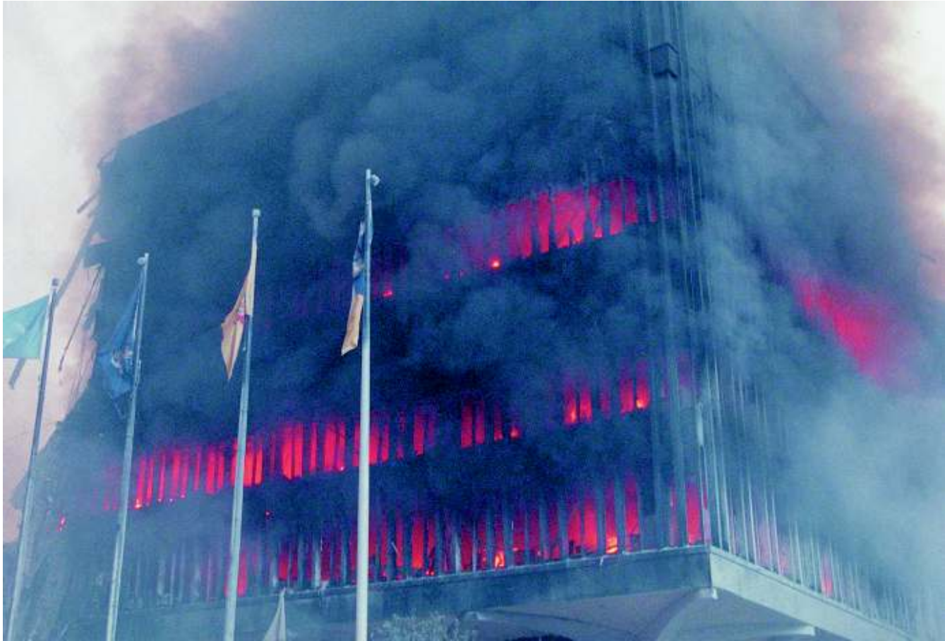
Figure 6-2 Both Buildings 5 and 6 suffered from extreme fires. These were “conventional” fires; i.e., giant flames were visible, even through dark smoke, and windows shattered.
