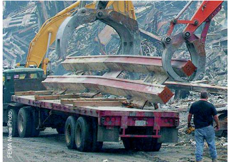
Figure 3-10 Two columns still attached to the three plates that made a pre-fab unit.
