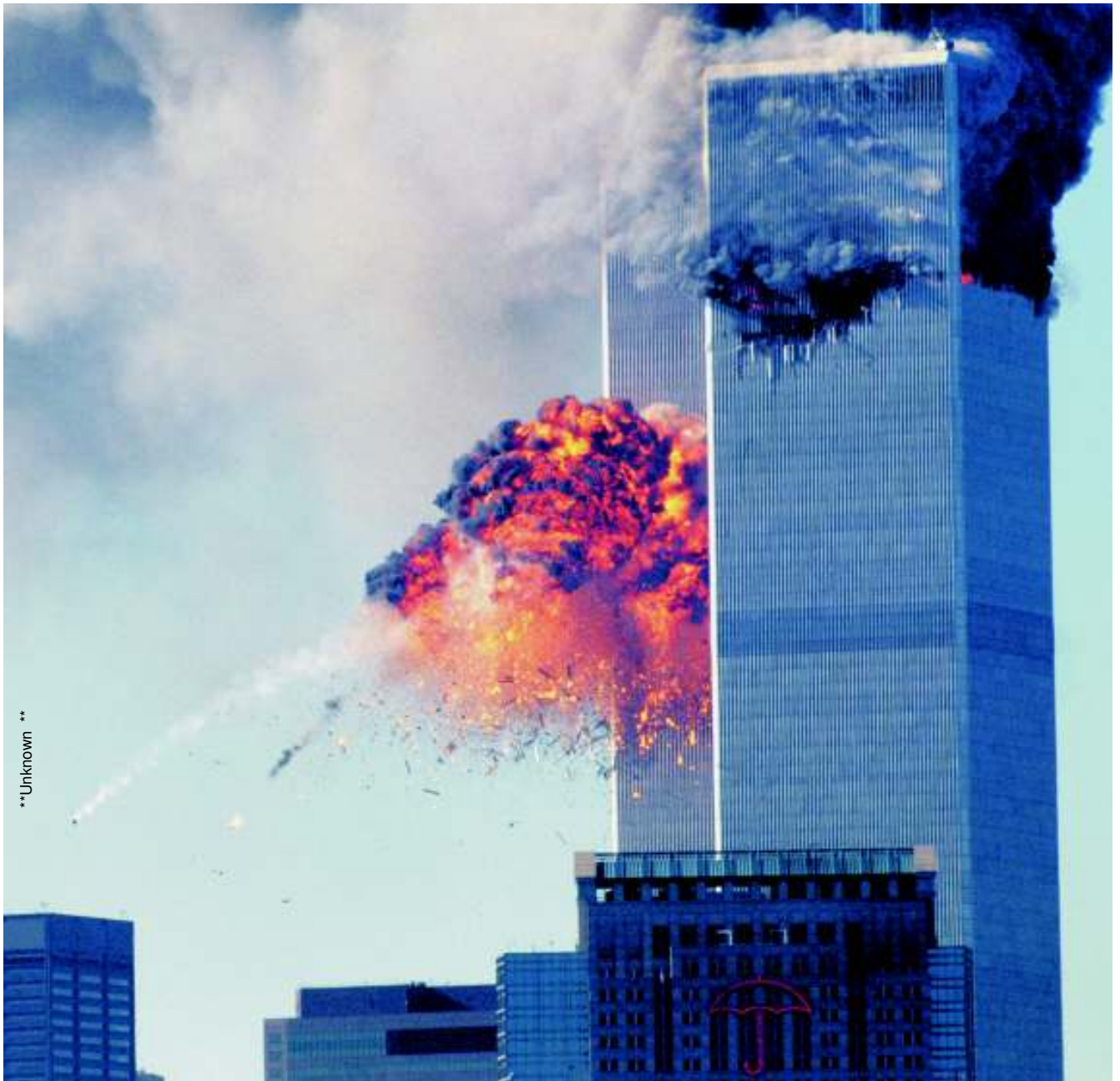
Figure 4-12 This photograph was taken slightly before the one in Figure 4-7. There are only a few flames in the North Tower, and the smoke is very dark. The fires have been burning for only 16 minutes but already most flames have vanished. Why didn't the fire grow over time?
