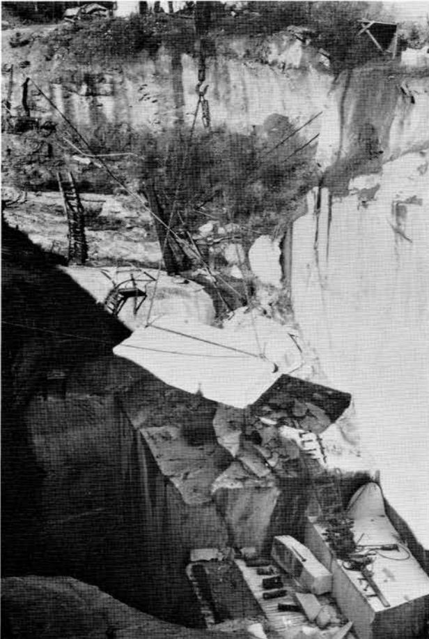
Quarrying was the most crucial phase of The Georgia Guidestones ® production because of the massive size of the granite slabs and the strain on men and equipment. It was accomplished in the more than 100-ft. depths of the "Pyramid Blue Granite" Quarry. "Our Quarry Superintendent, Jimmy Mattox, and his crew simply did a fantastic job under the circumstances," said Joe Fendley, builder of The Georgia Guidestones ® .
