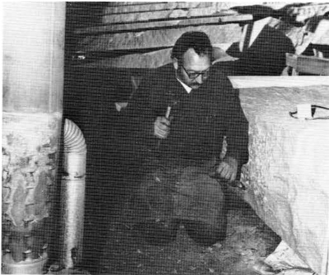
Horace Bradford, one of the two master stonecutters assigned to The Georgia Guidestones® project, is shown smoothing the sides of the center stone.
