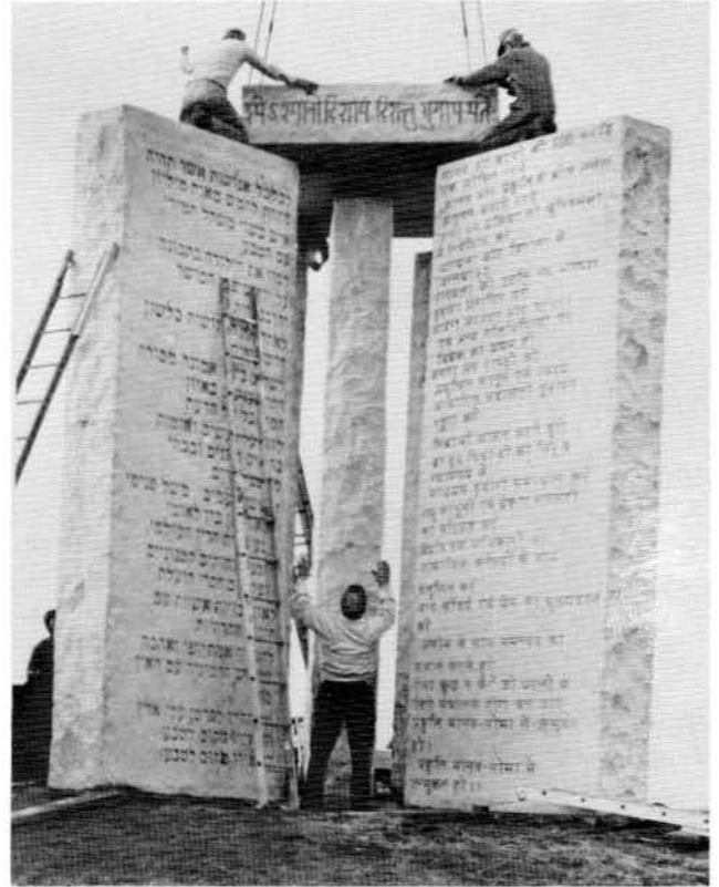
During the waning twilight of March 12, 1980 the final section, the large capstone, was set into place to complete construction of The Georgia Guidestones . Joe Fendley, builder, is shown directing placement of the capstone. All that remained to be done was steam-cleaning the stone for the March 22nd dedication.
