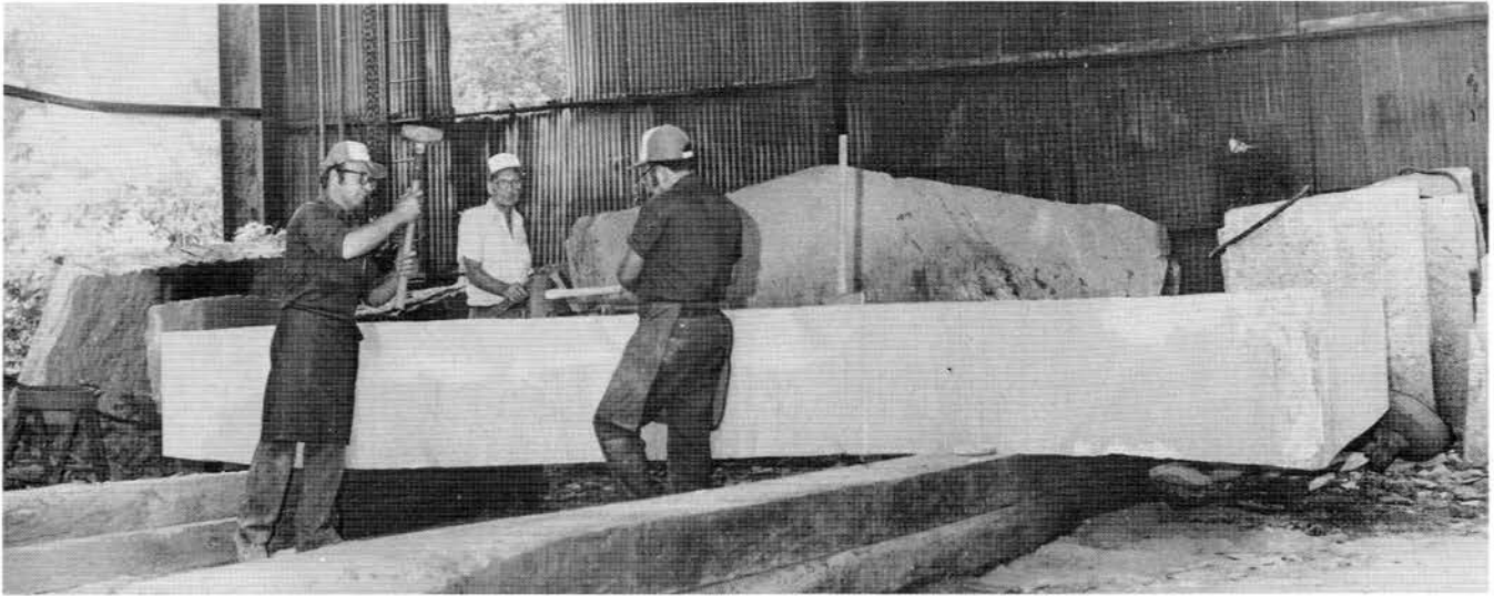
A special crew of Horace and Frankie Bradford, master stone craftsmen, under the direction of Joe B. Davis, background, a retired plant superintendent was hired to cut and pitch the granite slabs to the exact dimensions provided by "Mr. R.C. Christian." Special crews were hired because the project was so demanding that it would disrupt the regular Elberton Granite Finishing Company's production schedule.
