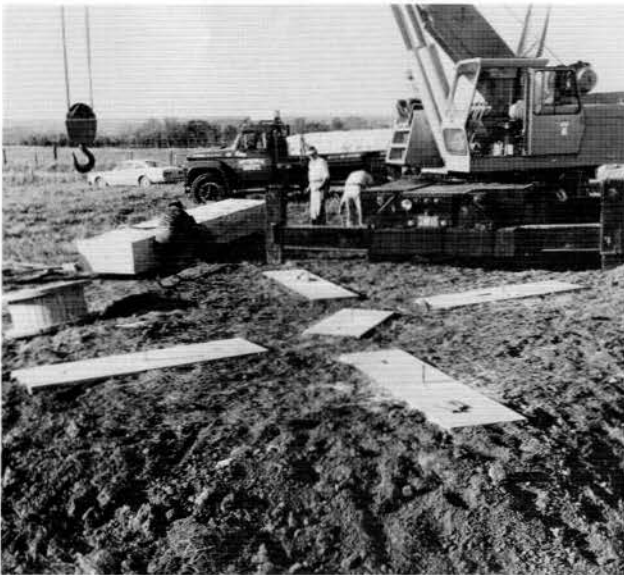
This photo shows the configuration of The Georgia Guidestones® four large outside base slabs, with a central or gnomon stone, arranged like a giant paddlewheel with the outer stones oriented to the limits of the migration of the moon during a year. The center stone is marked and holes drilled in it so that the sun rays mark the time of day and the seasons of the year. Also, the North Star is always visible through a special slot from the South to the North side of the center stone. An astronomer was employed to accurately achieve this placement of the stones.
