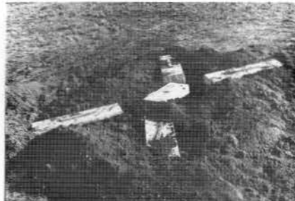
The base for The Georgia Guidestones® was set upon bed-rock and the giant "paddlewheel" is shown shortly after the concrete was poured.
