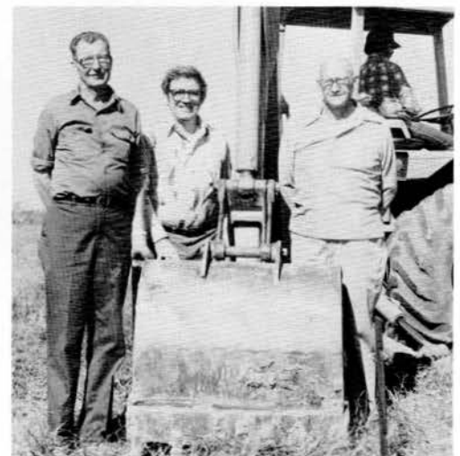
(l-r) Project superintendent Joe B. Davis, builder Joe H. Fendley, Sr., and foundation builder W.A. "Willie" Edwards pause during the early days of construction to pose for the camera.
