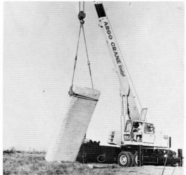
A Guidestone granite slab is shown being hoisted from the transporting truck by Grady Albertson, owner and operator of Argo Crane Service. This is the first of The Georgia Guidestones® to arrive at the erection site and its placement atop the foundation will mark history, for it is the first known "Message to Mankind" ever to be erected in the United States of America. Its purpose, as told by the sponsors, is to leave a message, etched in granite, that will survive the ravages of time.
