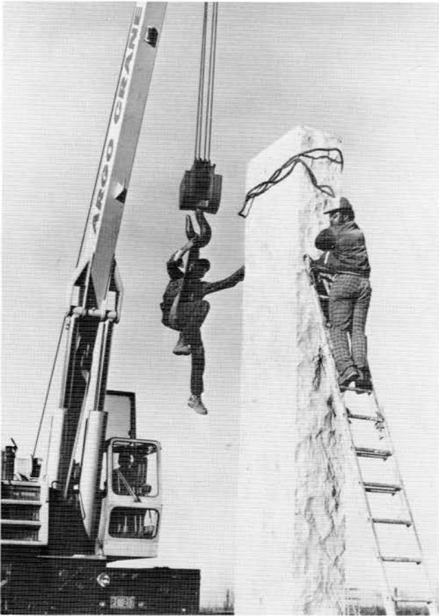
Workmen take cables loose as one of the Guidestones is placed in its rightful position. The rock-pitched finish on the sides is in accordance with "Mr. R.C. Christian's" instructions, that the finish conform as nearly as possible to the natural state of the granite as it is quarried.
