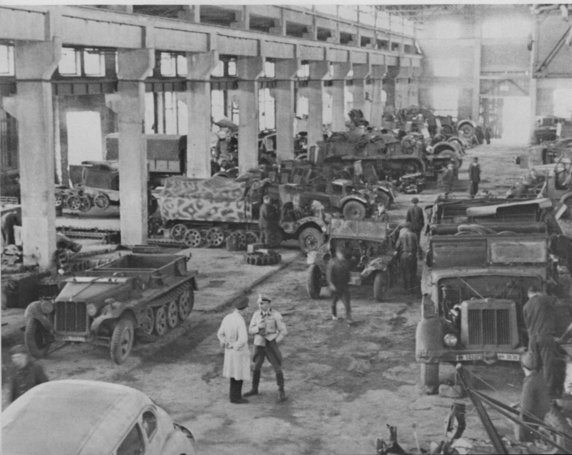
The pause that followed the completion of the Manstein Offensive allowed the repair of worn vehicles and the addition of new. [Left] A rare shot of a halftrack workshop, full of both Wehrmacht and SS vehicles in various stages of repair. From the left, the identifiable vehicles are a one ton, a three ton with Sand Yellow overspray with another one ton and an eight ton behind it, a one ton missing its hood in the center and a twelve ton to the right. Of interest is the difference in the pattern of the license plates on the twelve ton. [Bundesarchiv] [Above] This PzKpfw IV ausf F2 of Das Reich has also had its coat of Panzer Grey oversprayed with the newly authorized Sand Yellow. [Bundesarchiv]
