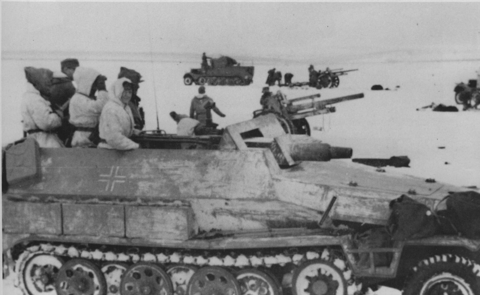
Passing in front of a field artillery battery, this "Stummel" of Leibstandarte makes an excellent study of the futility of temporary snow camouflage, wearing off almost completely where the engine or gun heat would melt snow or where the dismantling of the crew would rub it off. The Stummel [officially an SdKfz 251/9 mounting the 7.5 cm L/24 KwK], a brand new vehicle at this time, was extremely popular because it brought massive firepower to individual panzergrenadier companies. In the background are a pair of 10.5 cm IFH/18 Field Howitzers and a single SdKfz 11 three ton halftrack support vehicle. [National Archives]
