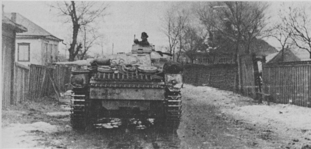
Passing in front of a field artillery battery, this "Stummel" of Leibstandarte makes an excellent study of the futility of temporary snow camouflage, wearing off almost completely where the engine or gun heat would melt snow or where the dismantling of the crew would rub it off. The Stummel [officially an SdKfz 251/9 mounting the 7.5 cm L/24 KwK], a brand new vehicle at this time, was extremely popular because it brought massive firepower to individual panzergrenadier companies. In the background are a pair of 10.5 cm IFH/18 Field Howitzers and a single SdKfz 11 three ton halftrack support vehicle. [National Archives]
