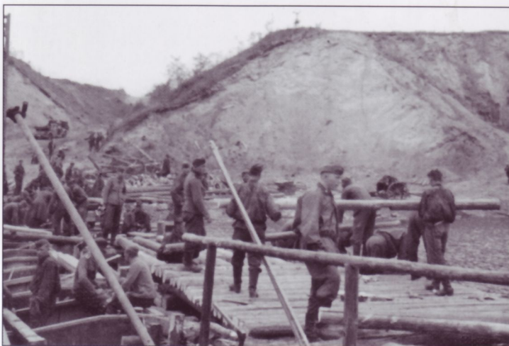
"Totenkopf" Division pioneers construct a bridge using local materials aided by locally confiscated boats. A timber bridge of this nature could only support comparatively light vehicles. This is an excellent location for a bridge.
