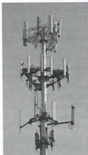
Figure 636: Gwen towers are installed across America and other countries.
