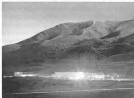
Figure 513: The multi-billion dollar 'data center' in Utah to filter and store global communications.
