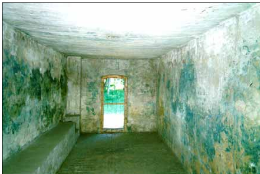
Photo 13: Delousing chamber in Stutthof, interior view from the south door. All walls exhibit the typical blue pigmentation due to iron cyanide.
