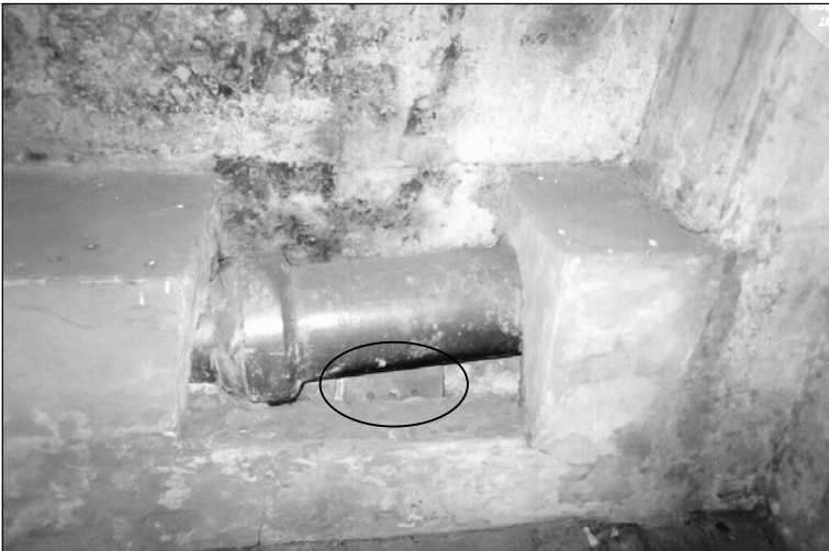
Photo 8: Delousing chamber at Stutthof, interior view, west wall; cast iron connection pipe to the oven located outside the delousing chamber and used to heat the air inside the chamber. The pipe was originally surrounded by masonry similar to that visible in the photograph, but of perforated brick. One of these bricks is still visible today, underneath and behind the pipe (circle). © Carlo Mattogno
