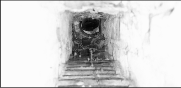
Photo 7: Delousing chamber at Stutthof, viewed from the south. The oven was used to heat the air inside the delousing chamber. Interior view of the combustion chamber. Beneath: the plane grid; above: the circular opening of the connection to the cast iron pipe located inside the delousing chamber. ©
