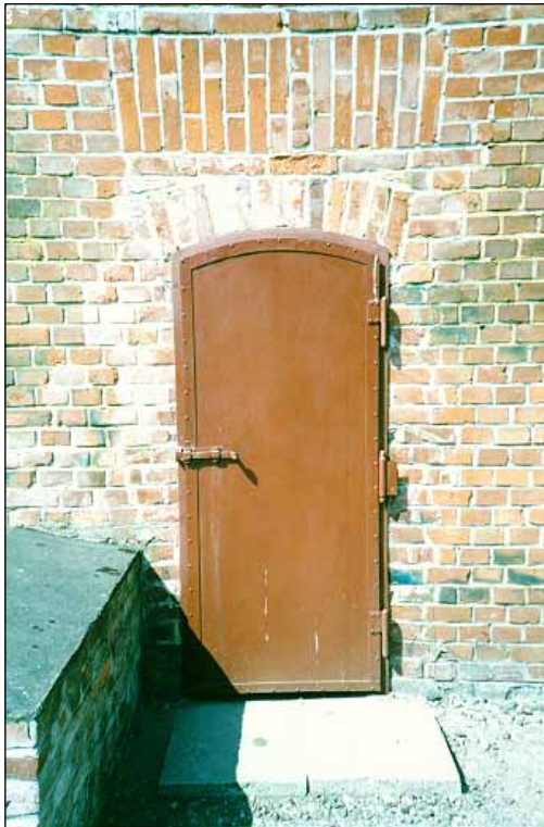
Photo 4: Delousing chamber in Stutthof, southeast side. The door today. It is not alleged that this was the original door. © Carlo Mattogno
