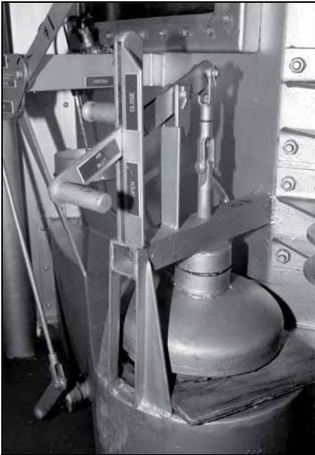
Fig. 84: Closeup of fresh air intake of gas chamber.
