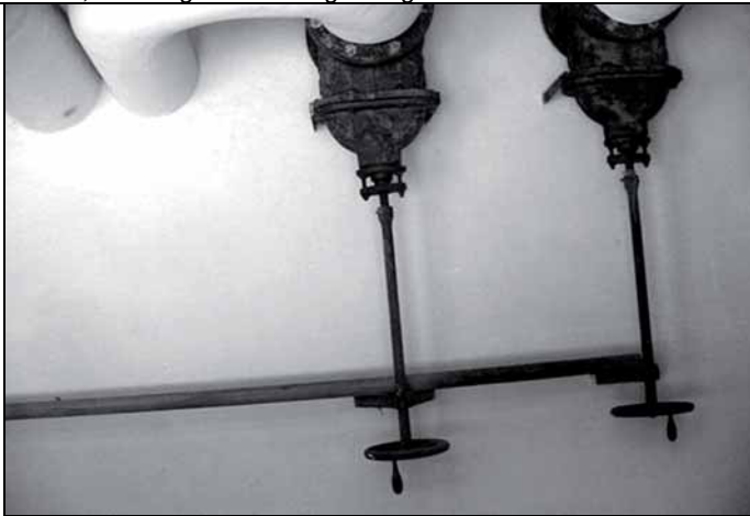
Fig. 51: Heavy insulated hot water (or steam?) pipes in the room behind the alleged gas chamber of Dachau camp, leading into the space above the current room. 1
