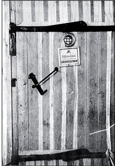
Fig. 25: Wooden disinfestation chamber door at Auschwitz rendered provisionally gas-tight with peephole and metal protection grid. This is what the gas-tight doors for the homicidal ‘gas chambers’ are supposed to have looked like. Note the extremely flimsy lock. 177
