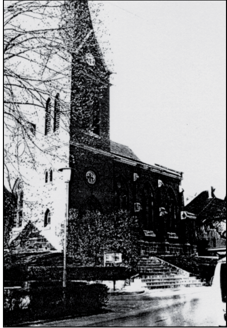
Fig. 36: In August 1976, the Protestant church at D-96484 Meeder-Wiesefeld was fumigated with Zyklon B. Subsequently, blue-colored stains appeared all over the plaster (see Fig. 37).
