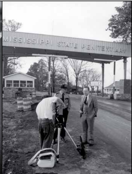
Fig. 99: Fred Leuchter and Major Bill Hoskins outside of penitentiary gate.
