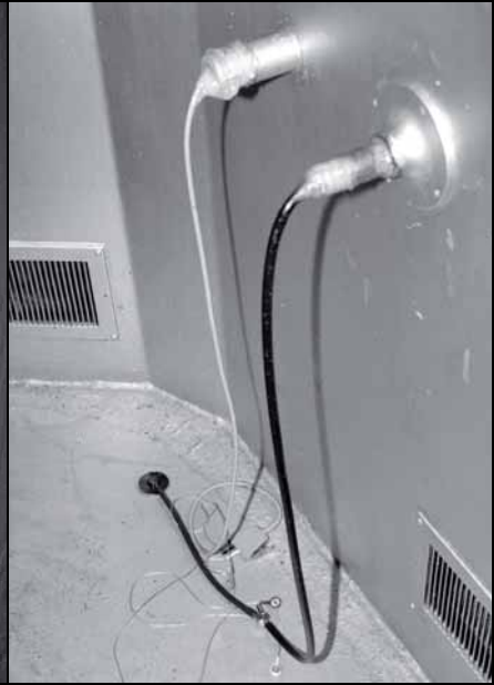
Fig. 97: Inside gas chamber where stethoscope and other body monitoring line enter. They are covered in vaseline to indicate leaks. Fresh air vents on the walls close to the floor.
