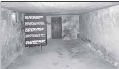
Fig. 40: Blue staining of the Zyklon B disinfestation installation, chamber III, of barrack 41 in Majdanek camp. (© C. Mattogno 202 )
