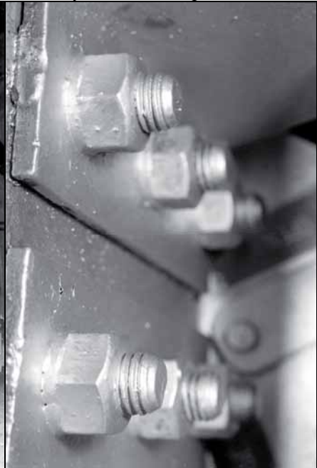
Fig. 95: Closeup of bolts on door hinges.
