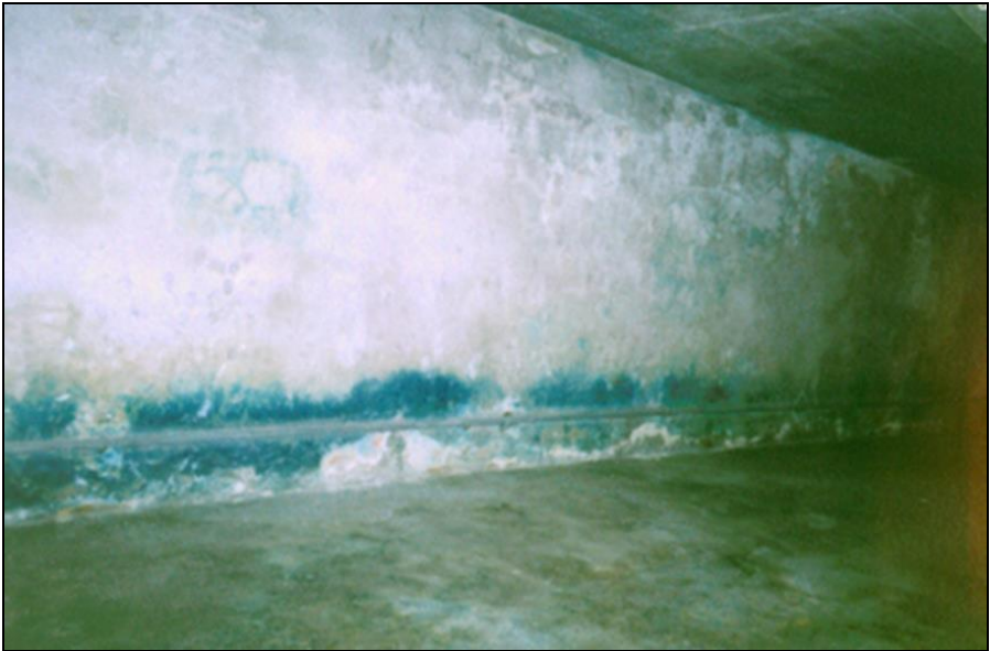
Photograph XIII: Disinfestation facility, Barrack 41, Chamber III, east wall. (© Carlo Mattogno.)
