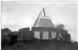
The Breaker's Head in Cedar Rapids, Iowa, has a very pointed roof. The pyramidal roof is made for a large Breaker's Head on the ground below. The Breaker's headroom, the place where the driver on and CEO meet.
