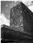
University Library (UNAM), Mexico City. Mexico, © W. Jacobson. In Architecture: A Visual History (© 2011) Architecture for Culture, Boston (design and Photo: Agnieszka
