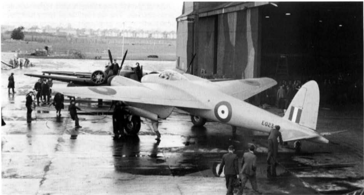
Bearing its original serial, E0234, the Mosquito prototype, painted bright yellow, is made ready for its first engine runs at Hatfield. The yellow paint scheme was intended to make the aircraft readily identifiable to British anti-aircraft gunners. (via Phil Jarrett)
