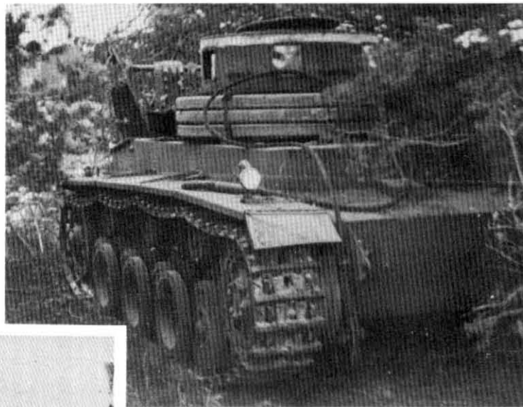
Plates 439-440. VK3001(H): left, with weights to simulate the turret; above, the chassis on trials.
