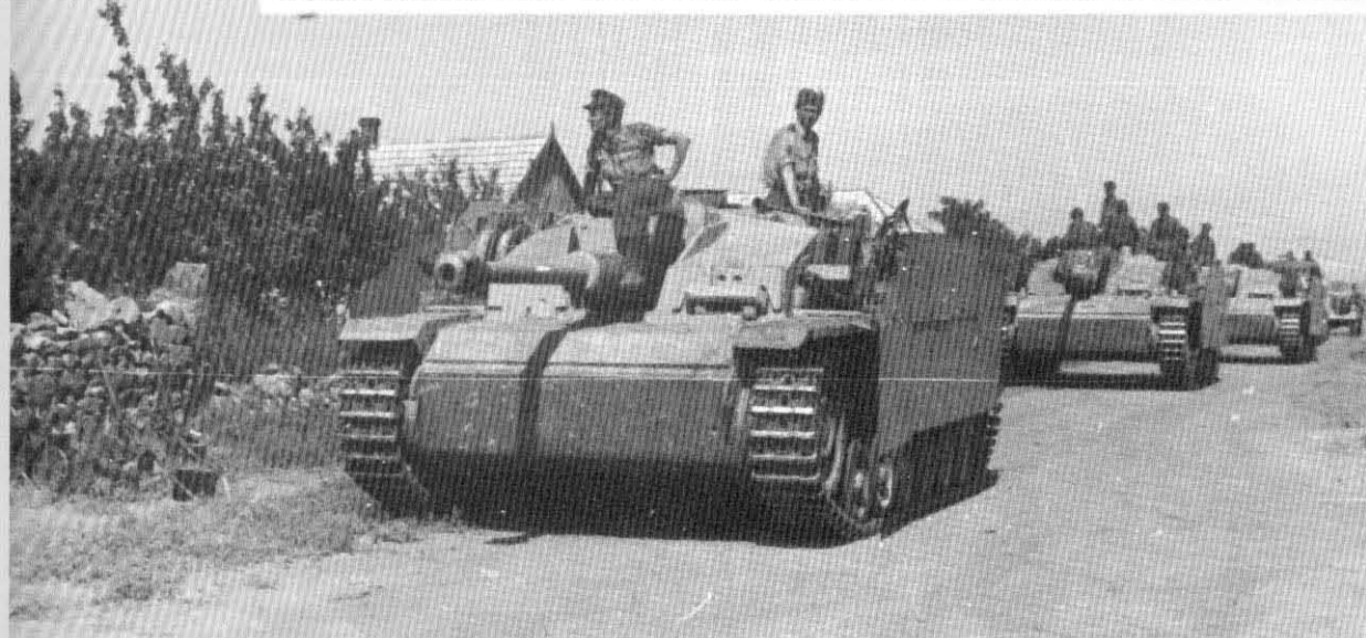
Plates 255-256. StuG III Ausf F/8. Note the additional armour on the front of the vehicle and the skirt armour.
