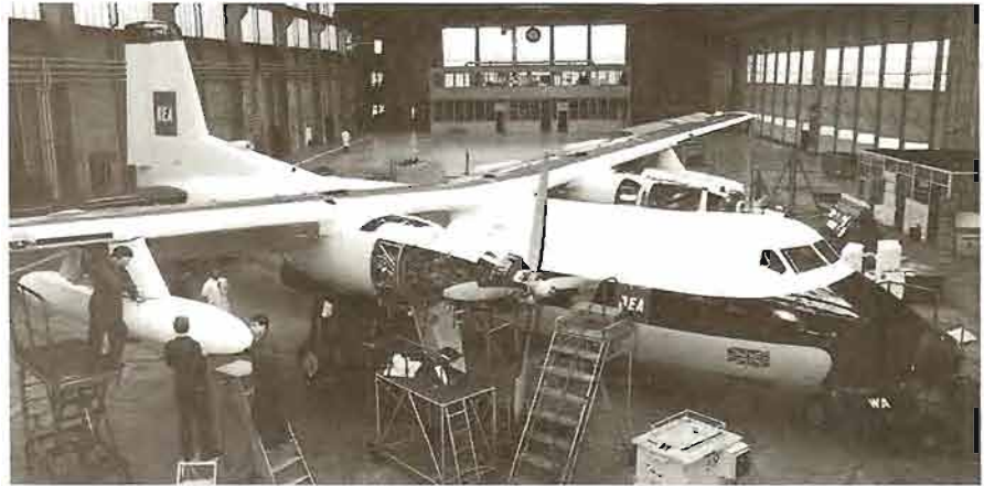
Above left: A Handley Page Herald of Air UK Above right: Captain J North and Flight Officer I Reed at the controls of a BEA Herald Above: Fitting long-range fuel tanks for a South American tour
