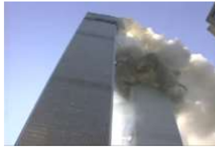
Destruction of WTC 2 on 9/11 in real life.
