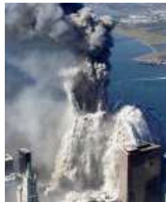
Steel “losing half its structural strength due to a fire started by burning jet fuel”
