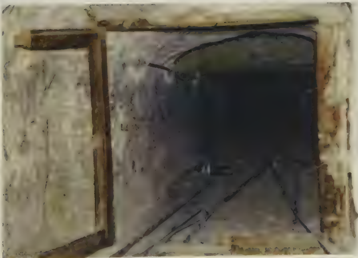
Plate 6. Niche opening: cover removed, looking in
