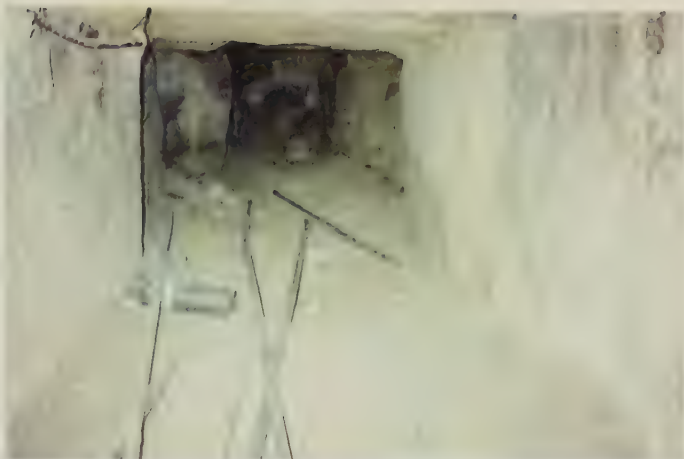
Plate 9. Photograph from inside the passageway, looking back toward the entryway
