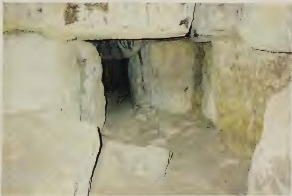
Plate 14. The tunnel's stonework, approaching the exit
