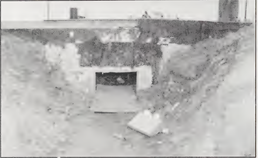
Underground bunker access assigned to Dave as seen following the siege after the Texas Rangers dug out the entrance. Note the sniper tower in the background (right), which kept him from leaving the ditch.
