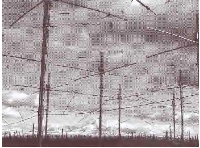
Figure 242: Some of the technology at the HAARP project in Alaska
