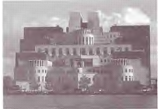
Figure 152: The overseas intelligence service, MI6, has a building alongside the River Thames that has the feel of a pyramid with the capstone missing
