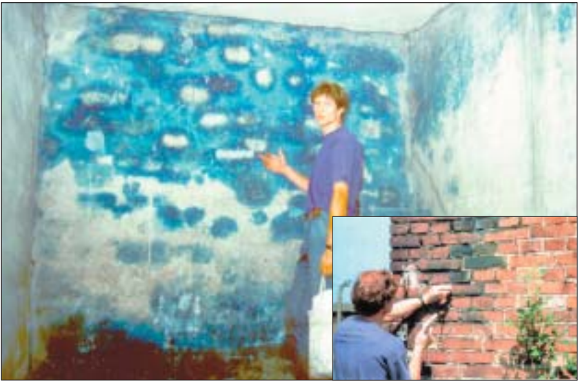
Color Image 3: Northwest room of the Zyklon B disinfestation wing of BW 5a in the Auschwitz-Birkenau camp. The external walls (background and to the right) show an intensive blue discoloration caused by the application of Zyklon B (HCN). The internal wall to the left was added later and is therefore free of cyanide residues. Color Image 4 (inset): Exterior of a wall of the same part of BW 5a. Cyanide penetrated the wall and caused blue stains.
