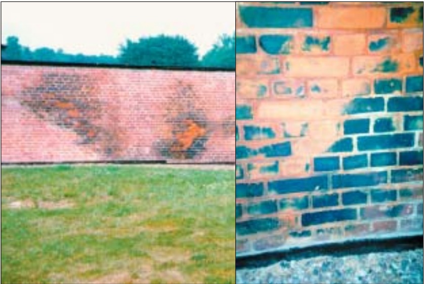
Color Image 10 (left): Blue discoloration of the east exterior wall of the Zyklon B disinfestation installation in the Stutthof camp. Color Image 11 (right): section enlargement. © C. Mattogno
