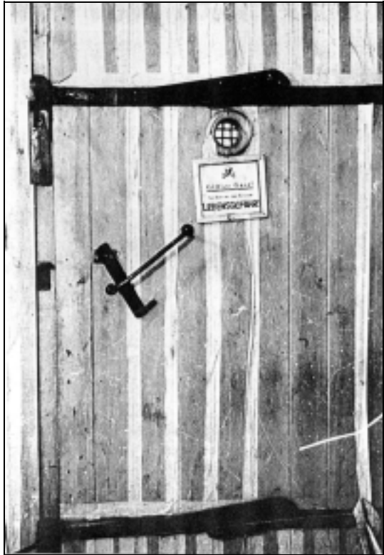
Fig. 33: Wooden disinfestation chamber door at Auschwitz, rendered provisionally gas-tight with peephole and metal protection grid. This is what the gas-tight doors for the homicidal ‘gas chambers’ are supposed to have looked like. Note the extremely flimsy lock.
