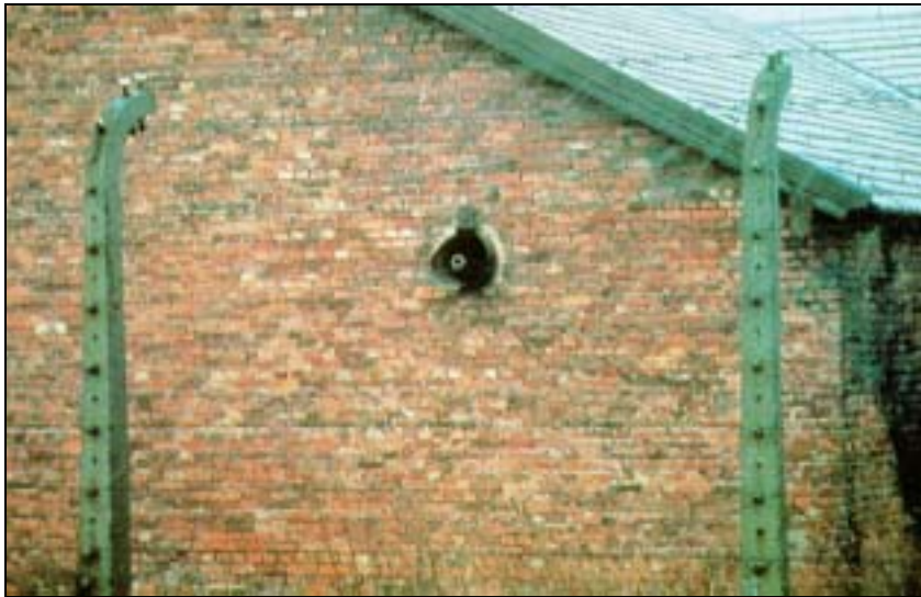
Fig. 19: Ventilation outlets from the disinfestation wing of building BW 5b, without equipment today. The ends of the water pipes are visible inside; see also Fig. 20.
