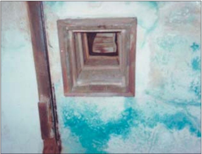
Color Image 6: Blue discoloration of the ceiling of the large Zyklon B disinfestation chamber, barrack 41 in Majdanek camp (Bad und Desinfektion I), caused by the application of Zyklon B. © C. Mattogno
