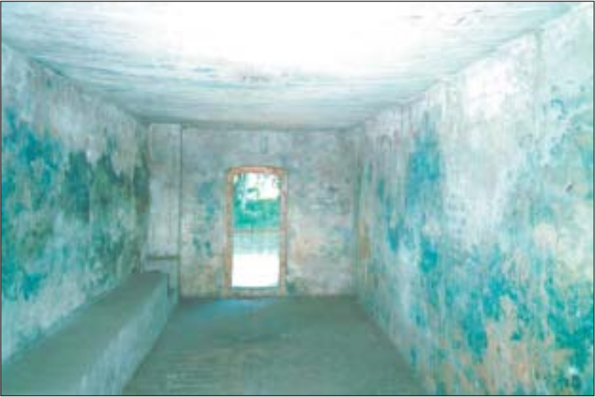
Color Image 9: Blue discoloration of the interior walls of the Zyklon B disinfestation installation in the Stutthof camp. © C. Mattogno
