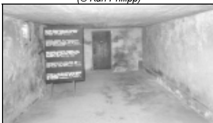
Fig. 61: Zyklon B disinfestation installation, chamber III, of barrack 41 in Majdanek camp. (© C. Mattogno 316 )
