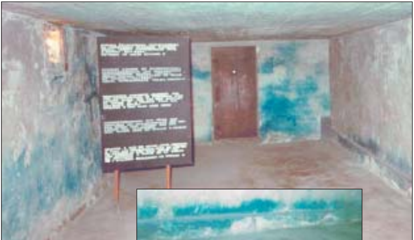
Color Image 7: Blue discoloration of the interior of the walls of chamber III, disinfestation installation barrack 41 (Bad und Desinfektion I) in Majdanek camp, caused by the application of Zyklon B. Color Image 8 (inset): East wall of this chamber. © C. Mattogno
