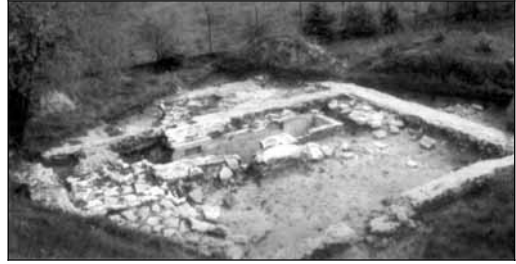
III. 95: Photo of the ruins of a garage building with repair pit in Belzec. 721
