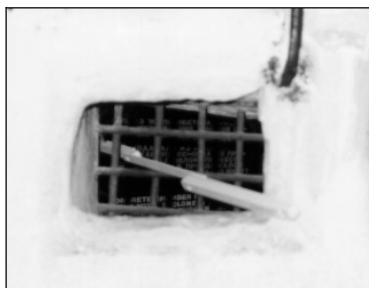
III. 100: Barred opening in the wall of room I in disinfection building 41, Majdanek camp (cf. plan section III. 99)
