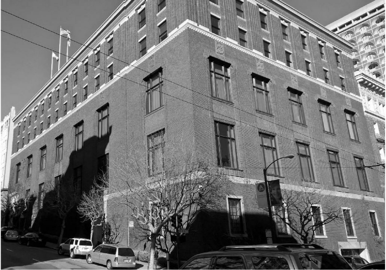
The headquarters of the Bohemian Club at the corner of Post and Taylor streets in San Francisco. There is also a second headquarters at Bohemian Grove in Sonoma County.
