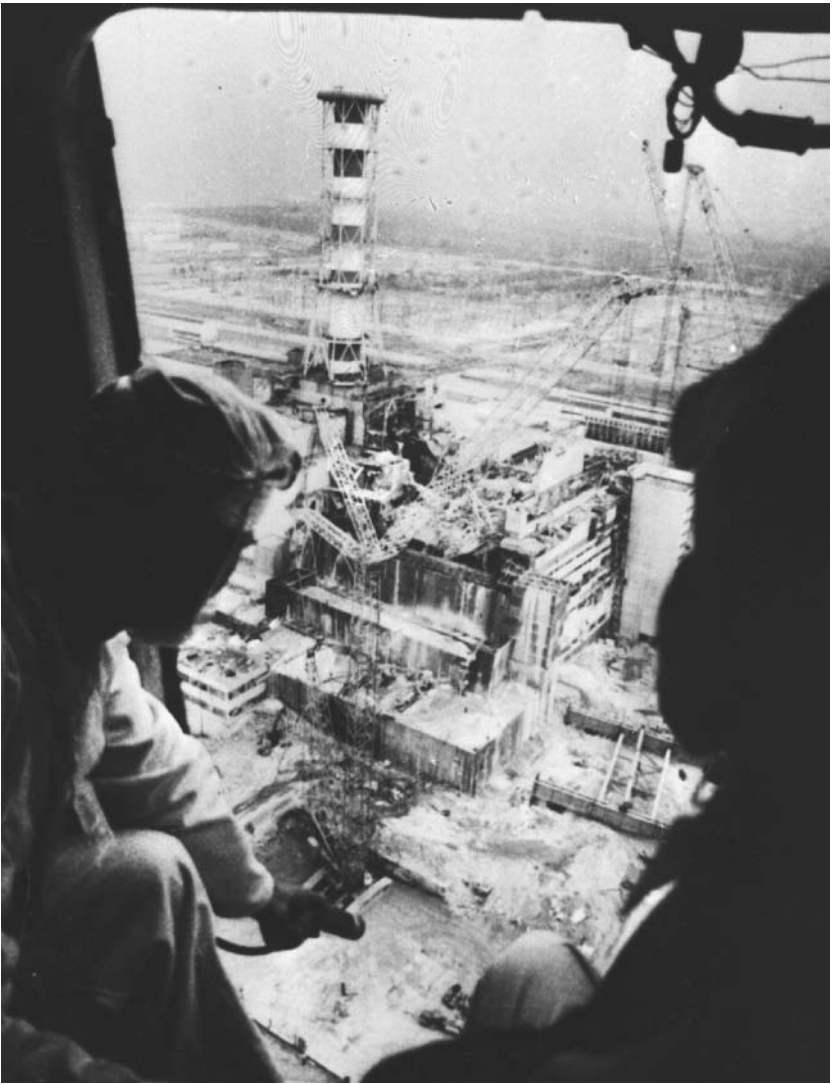
The destroyed reactor after the explosion and fire as seen from the open door of a helicopter.
