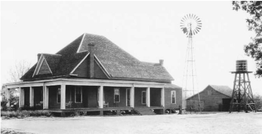
The windmill in the background at this farm home is used to drive a water pump that brings well water to the surface. (Courtesy of the Agricultural Research Service)
