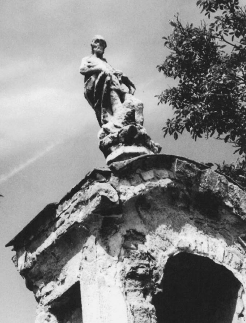
Acid rain attacks many materials. Limestone, a common material used by masons and sculptors, is particularly vulnerable. At one time, this limestone tomb was capped by a fine sculpture, but the stone has now eroded to a ruin. (Courtesy of Alexander Murashov, East Carolina University)
