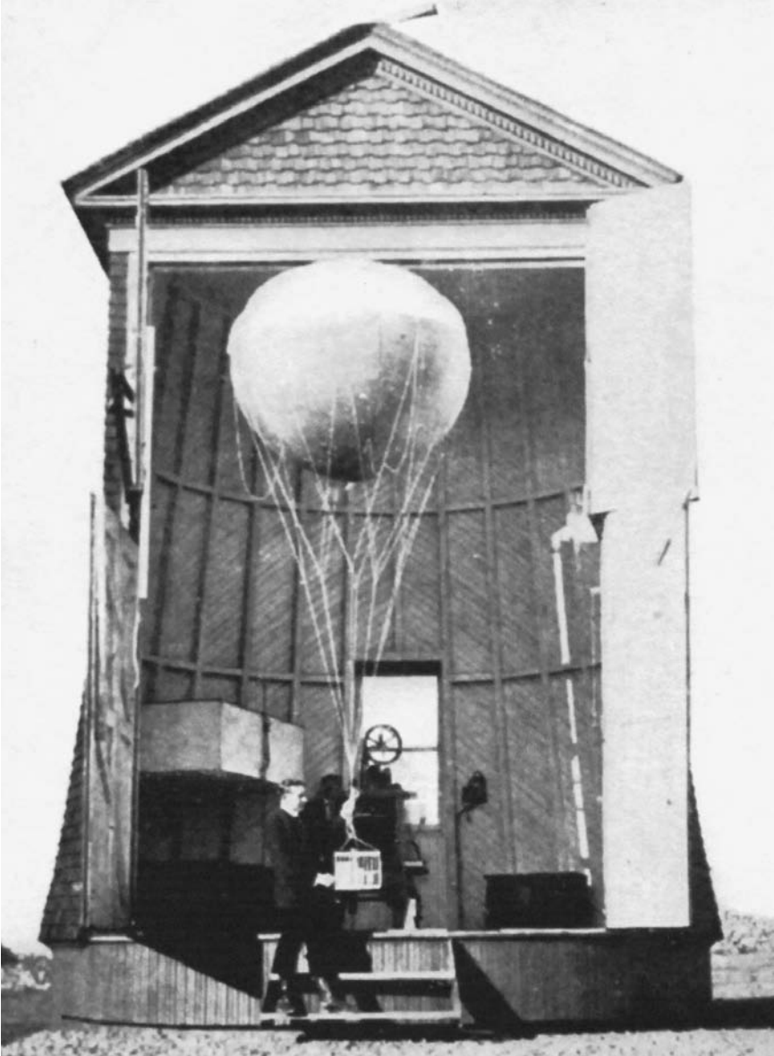
This photograph of a weather balloon-launching platform was taken about 1906. (Courtesy of the National Oceanic and Atmospheric Administration)
