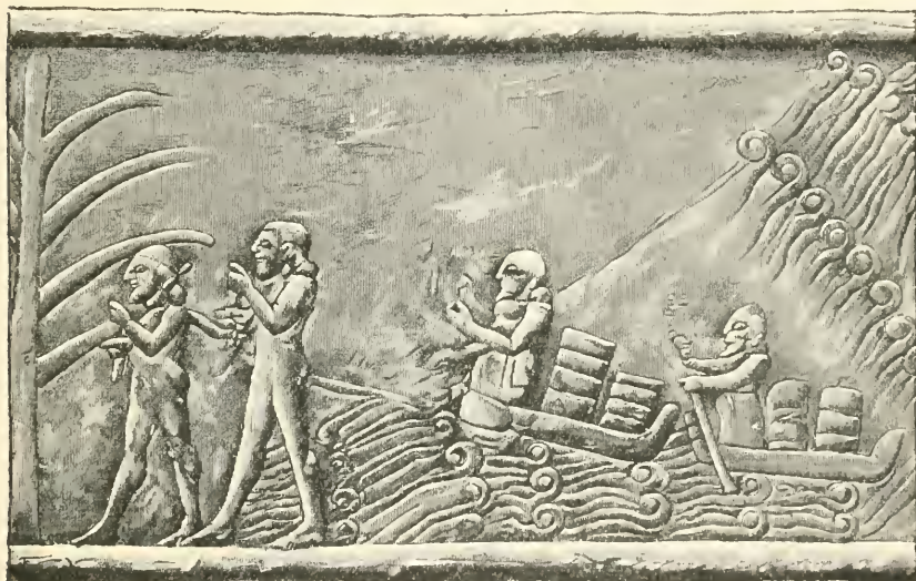
TRANSPORT OF BUILDING MATERIALS BY WATER. 2
