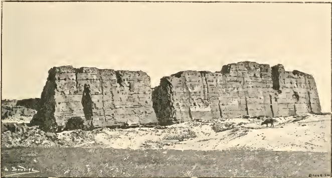
ONE OF THE FAÇADES OF THE FORTRESS OF KUBBÂN. 2
