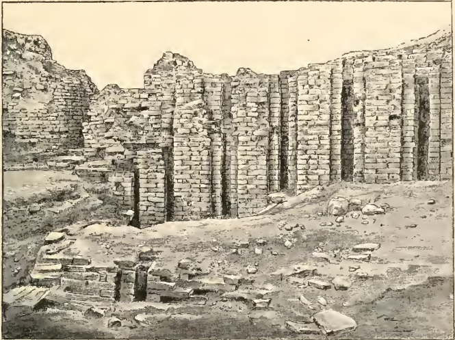
MILASTERS ON THE FAÇADE OF GUDEA'S PALACE. 2
