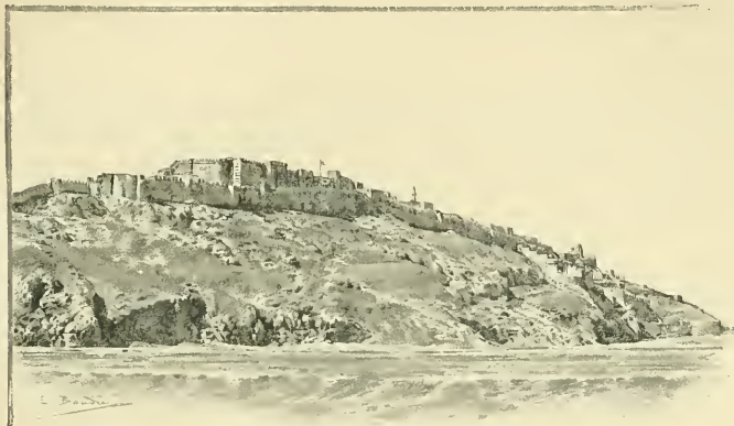
ENTRANCE TO THE MODERN CITADEL OF VAN FROM THE WESTWARD. 2
