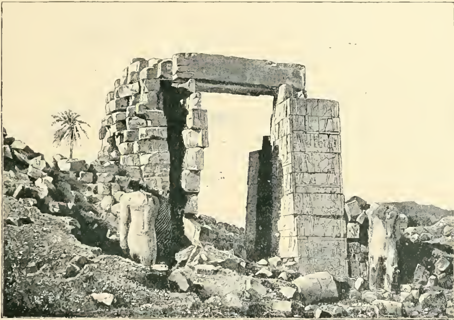
THE FIRST PYLON OF HARMHABÎ AT KARNAK. 1
