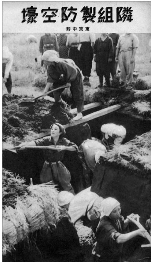
22-24. PWR 136, 2 October 1940, pp. 6-7. "The Neighborhood Association Bomb Shelter, Nakano, Tokyo." The women's brigade builds an air shelter under the supervision of Mr. Fujii, who shows them how to make the measurements and use shovels. Evidently, these women can spare ten hours in one day and perform hard manual labor.
