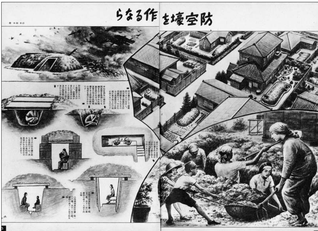
38. PWR 184, 3 September 1941, pp. 4-5. "How to Build an Air Raid Shelter." The responsibility for air defense fell heavily upon women. These are government instructions for building a backyard air raid shelter. It is dug, fortified, and operated by women, with the assistance of children, not men. The artist was one of Japan's best-known illustrators, Suzuki Gyōsui.
