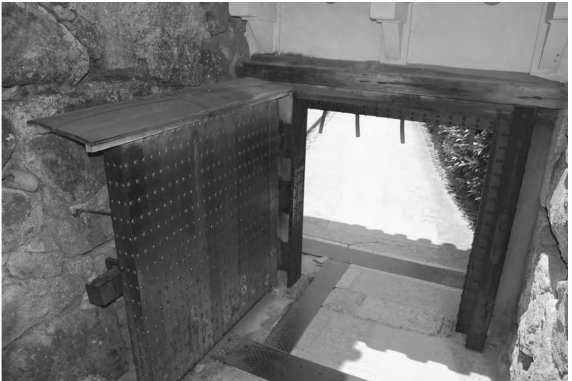
10.7 The Ho Gate of Himeji Castle leads to the entrance of the First Water Gate, which is the most direct route to the main tower ( tenshu ). One of many gates that soldiers would encounter en route to the castle, these fortifications were designed to confuse as well as to protect. The iron plating on the gate door provided additional means of defense. (Photo William E. Deal)
