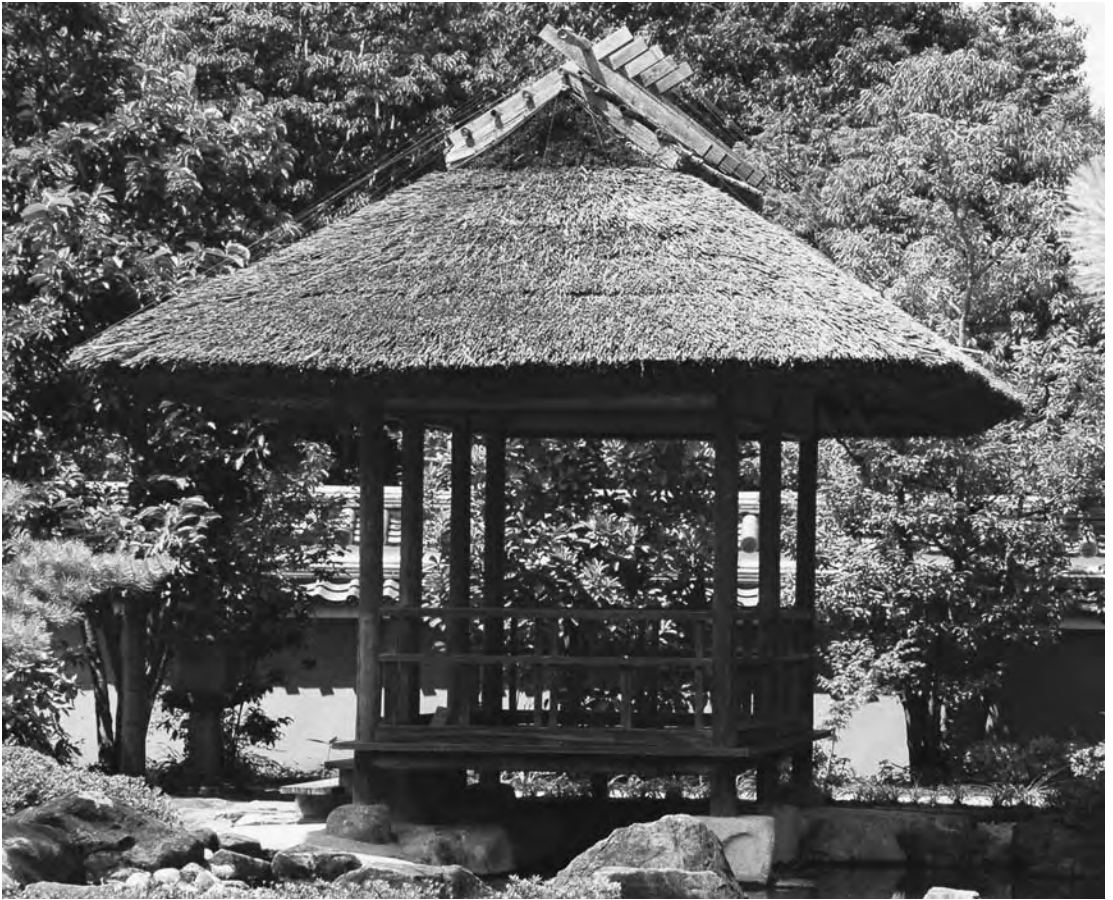
2.2 Example of the use of thatch in roof construction (Photo William E. Deal)
