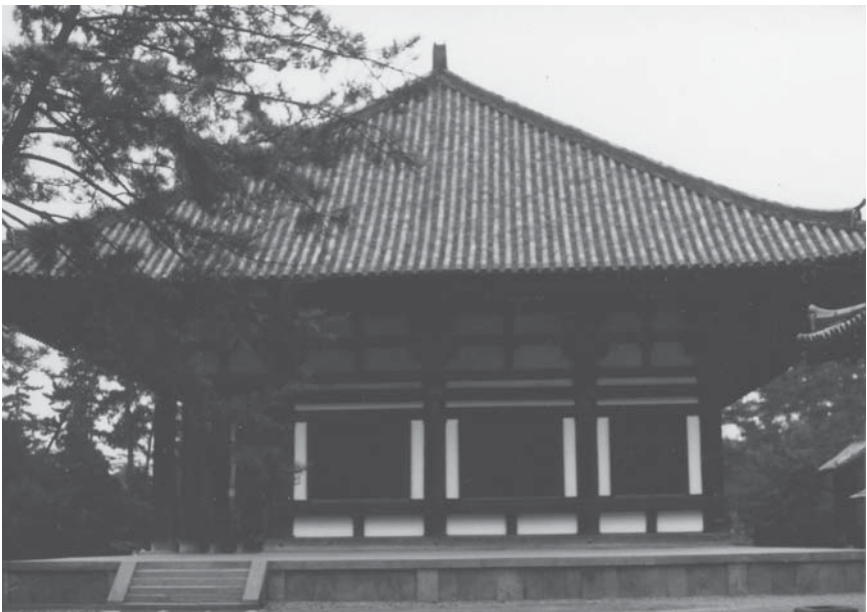
Nara: Toshodaiji temple Kondo, built by blind monk Ganjin, in traditional Chinese Tang Dynasty architecture
