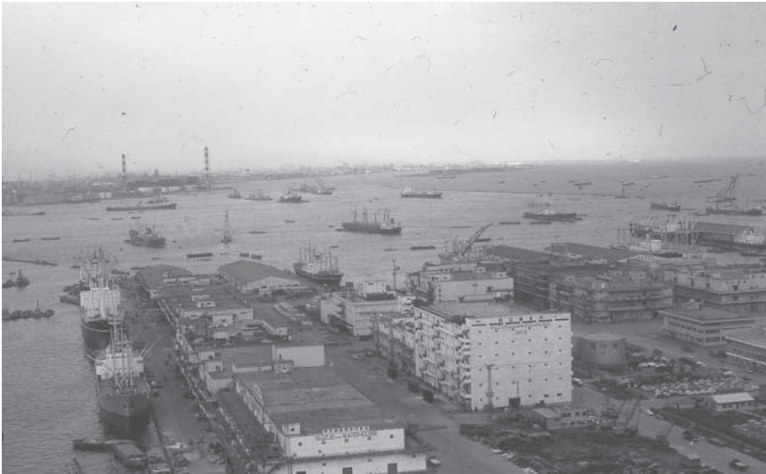
Modern Yokohama harbor, approximate site of Perry's landings and treaty
