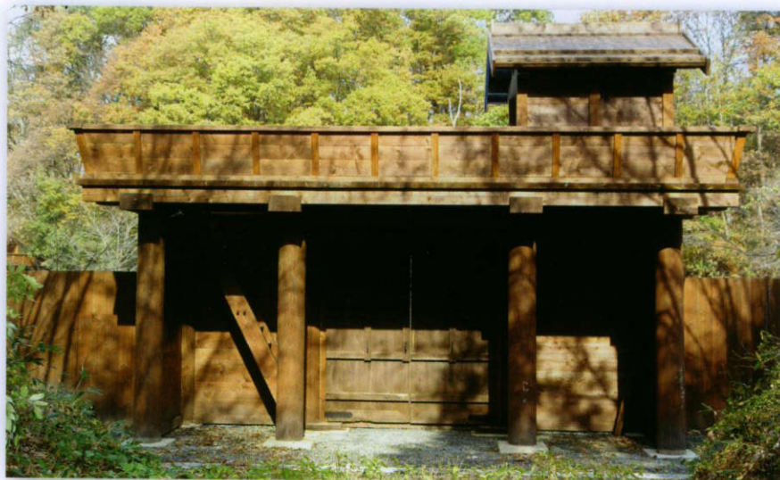
This useful reconstruction at the Esashi Fujiwara Heritage Park is an attempt to recreate the main gateway of Abe Sadatō's Kawasaki Castle, the site of much fighting in 1057 during the Former Nine Years' War. It is made completely from wood, with sloping parapets and a small guardhouse.
