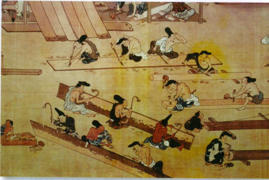
Several techniques used by Japanese carpenters in the construction of wooden castles are shown here in this scroll on display in the Ichijōdani Historical Museum near Fukui. In the bottom right a cutting line is being marked along a piece of timber using ink. Six men use adzes to smooth cut timber, while in the background more highly skilled carpenters produce the final finish using sharp blades.
